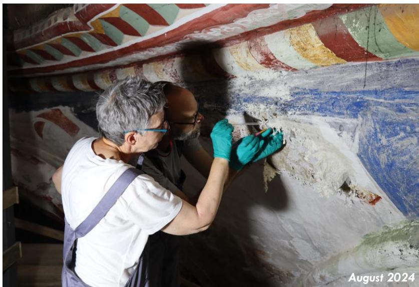
Images above: The Church of the Virgin, main space, north-west pendentive. Treatment processes: facing with lens tissue and Paraloid B72®, grouting and reinforced with pressed.
