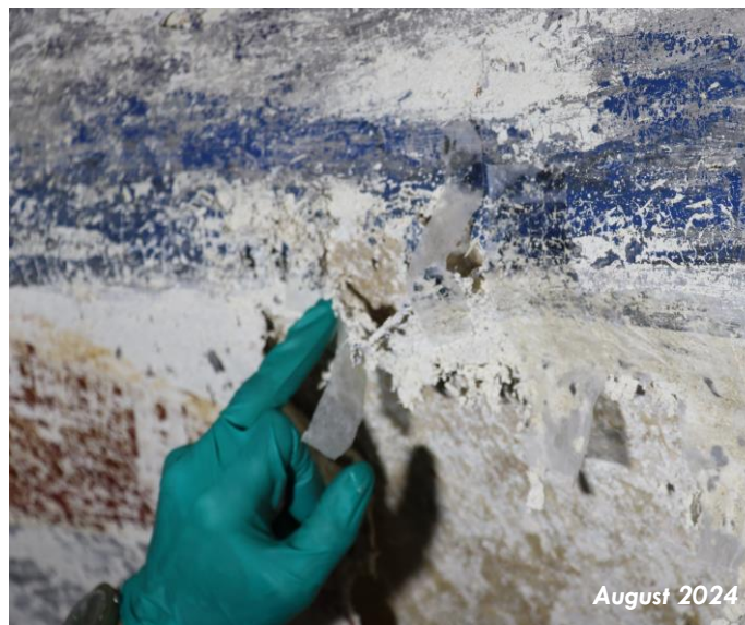
Images above: The Church of the Virgin, main space, north-west pendentive. Treatment processes: facing with lens tissue and Paraloid B72®, grouting and reinforced with pressed.
