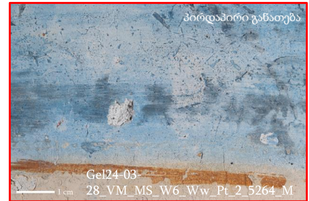
Right: damaged area sampled for further studies.
