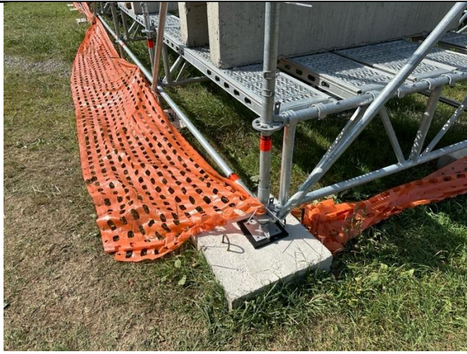
Description: Technical Control of Scaffolding
