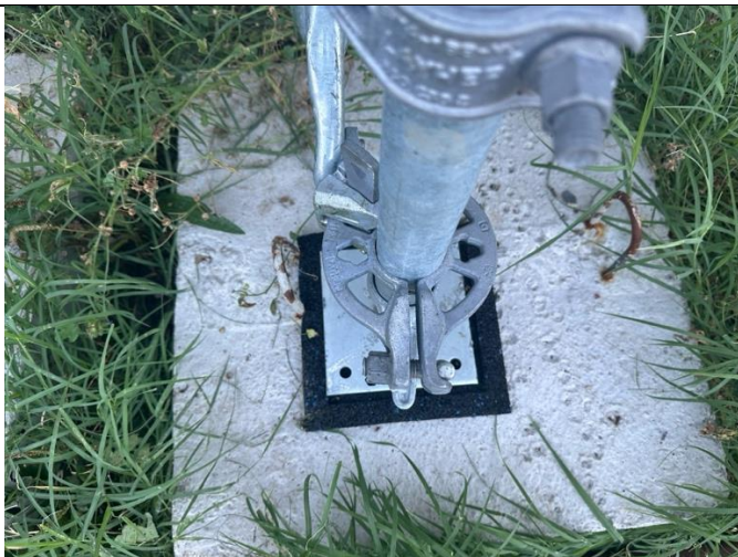
Description: Technical Control of Scaffolding
