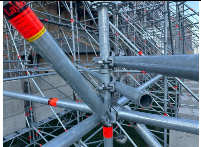
Description: Technical Control of Scaffolding
