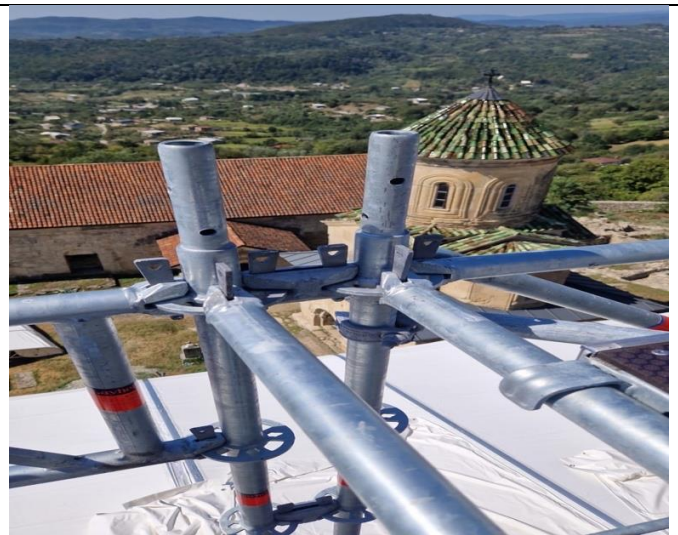
Description: Technical Control of Scaffolding
