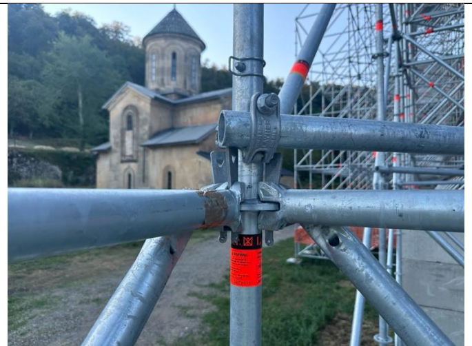
Description: Technical Control of Scaffolding
