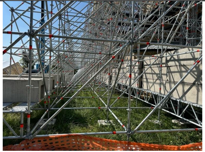
Description: Technical Control of Scaffolding
