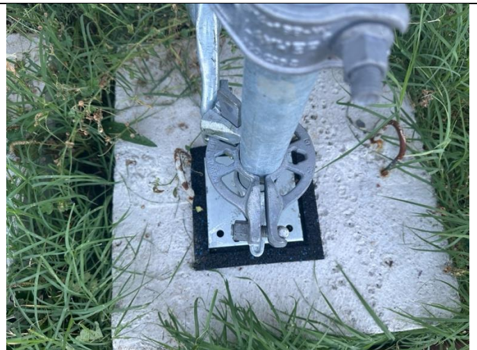
Description: Technical Control of Scaffolding
