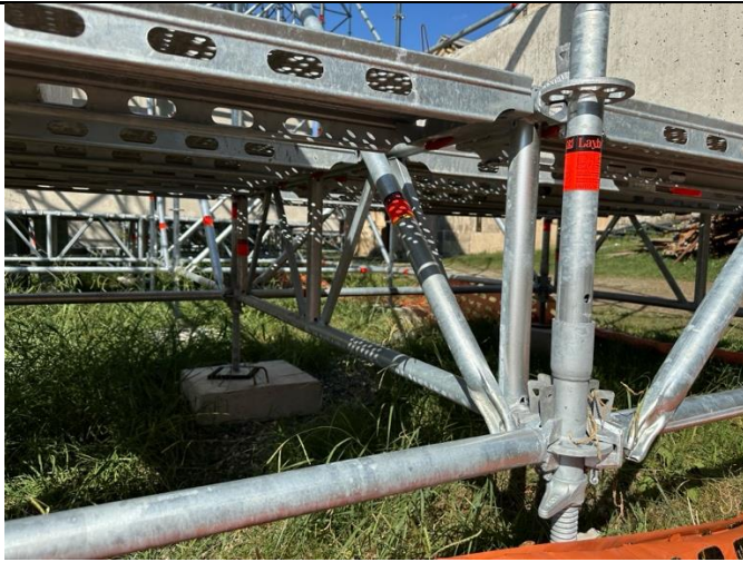
Description: Technical Control of Scaffolding
