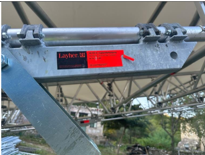
Description: Technical Control of Scaffolding
