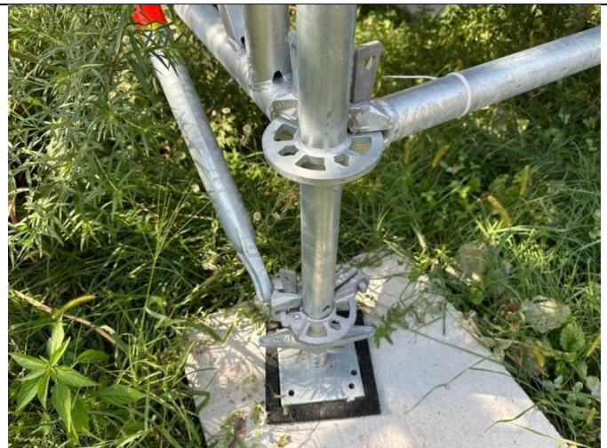
Description: Technical Control of Scaffolding
