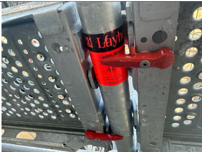
Description: Technical Control of Scaffolding
