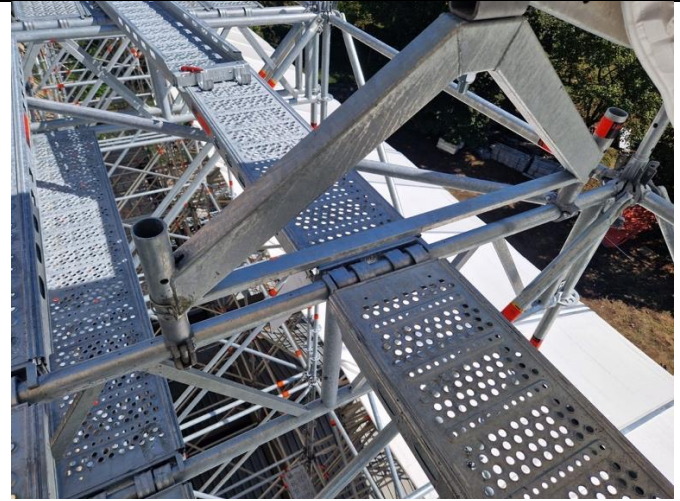
Description: Technical Control of Scaffolding
