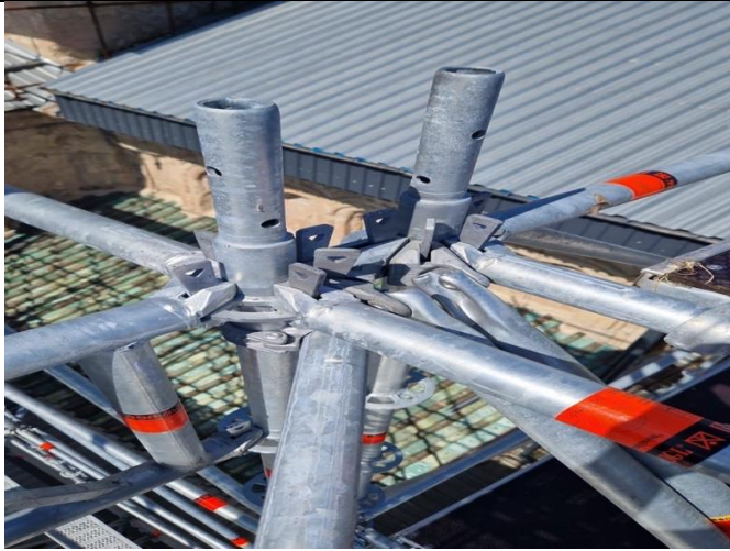
Description: Technical Control of Scaffolding
