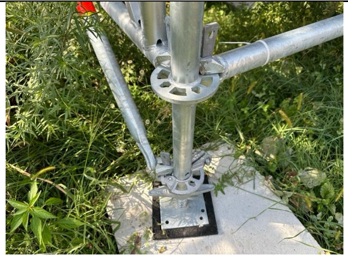
Description: Technical Control of Scaffolding
