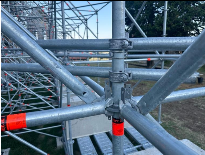
Description: Technical Control of Scaffolding
