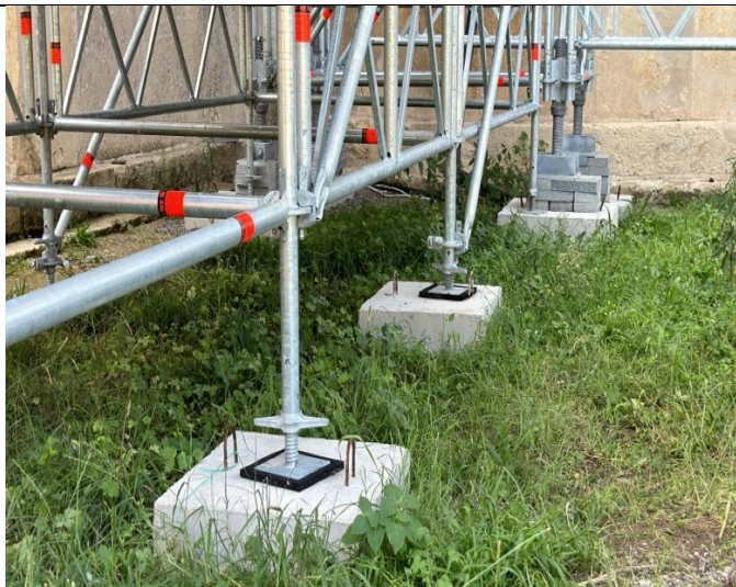
Description: Technical Control of Scaffolding
