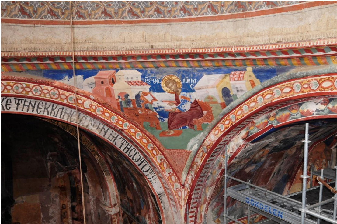
Fig. 11. S-E pendentive: existing condition.
