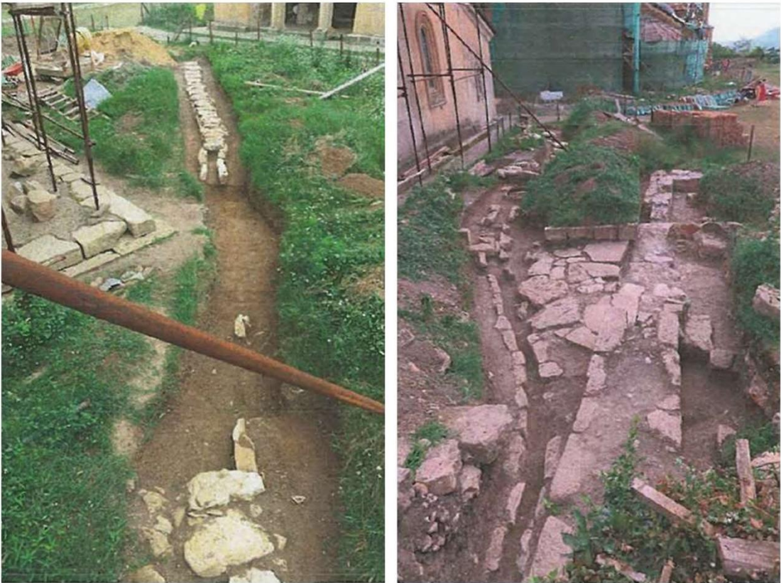
Fig. 15. Photo documentation of drainage collector in the Monastery grounds near the churches.
