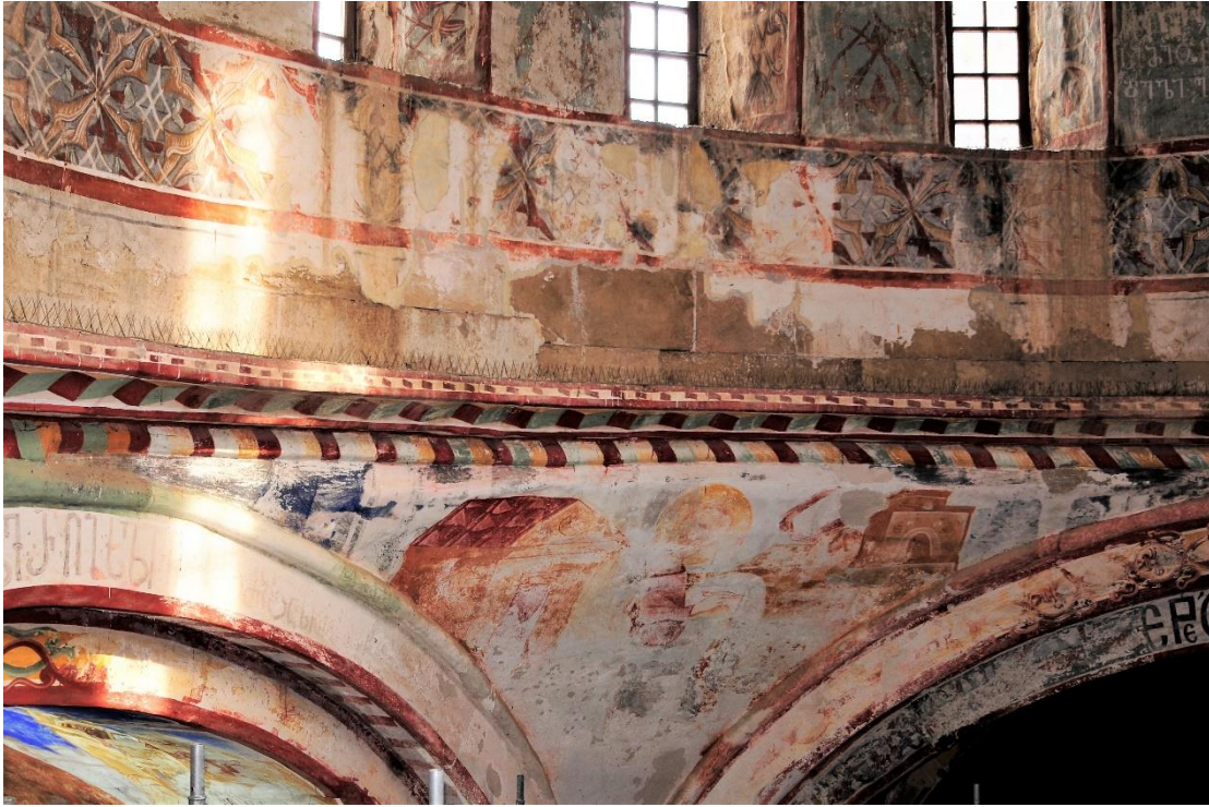
Fig. 10. N-E pendentive: moisture effects.
