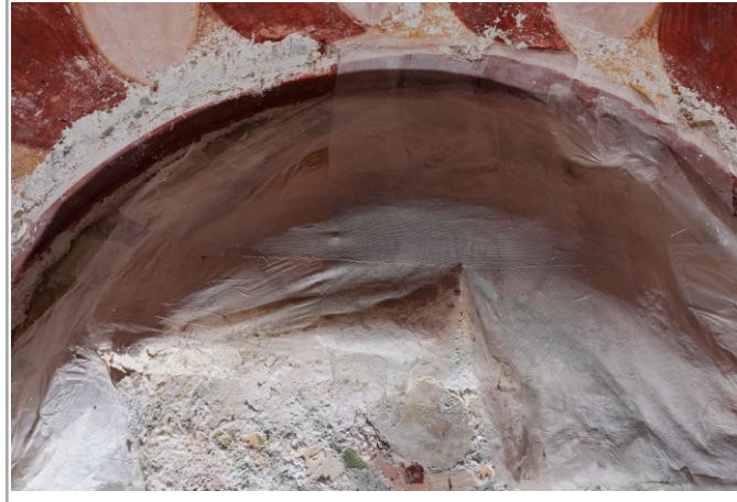
Two months after reinforcement. May 2024
