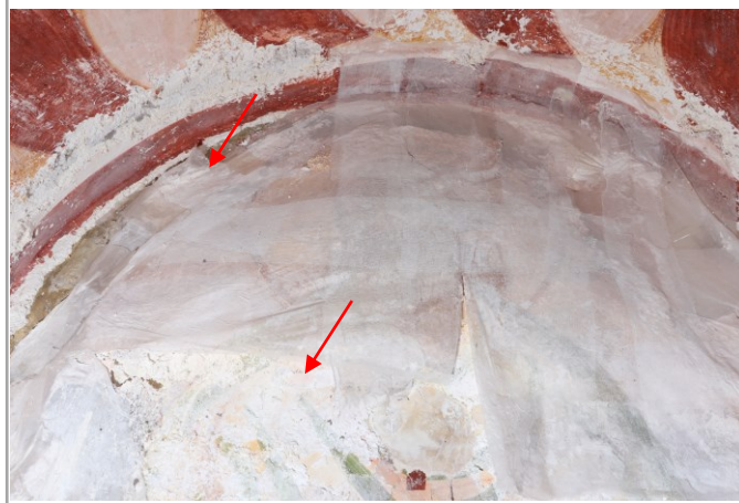
Two months after reinforcement. May 2024
