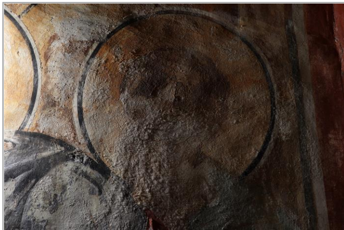
Before salt removal
