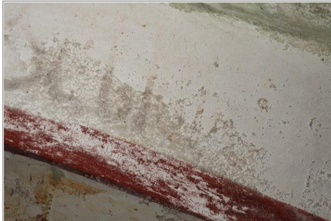
Before salt removal
