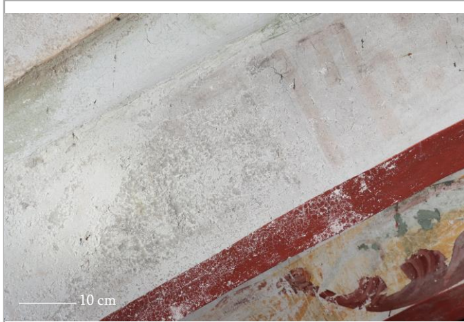
Before salt removal
