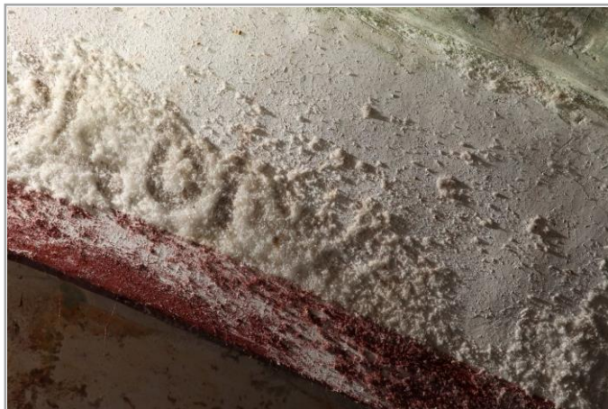
Before salt removal
