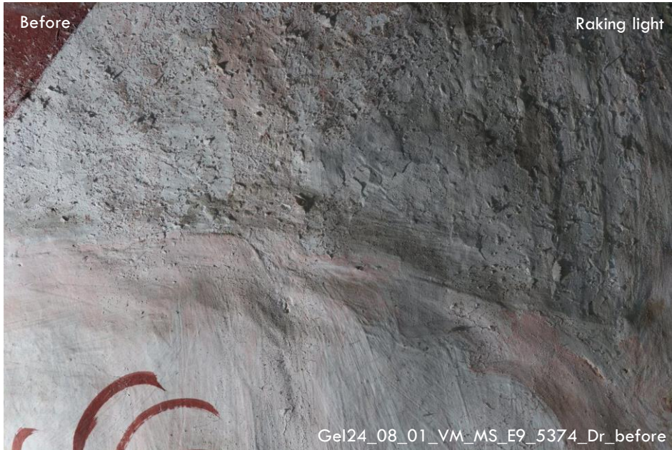
Above Condition of wall paintings before intervention in August 2024. The paint layer is flaking.
