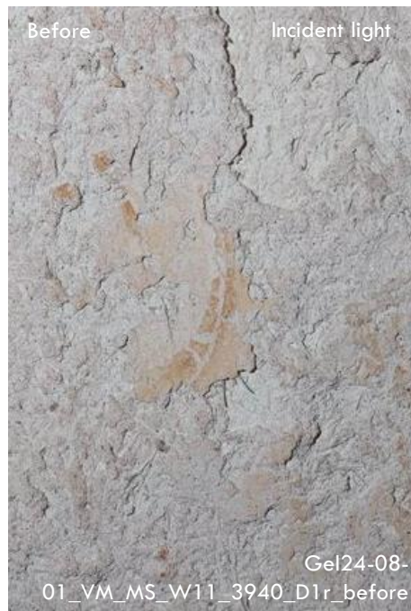
Above: Condition of wall paintings before intervention in August 2024. Plaster delamination, plaster powdering, exposed plaster edges;
