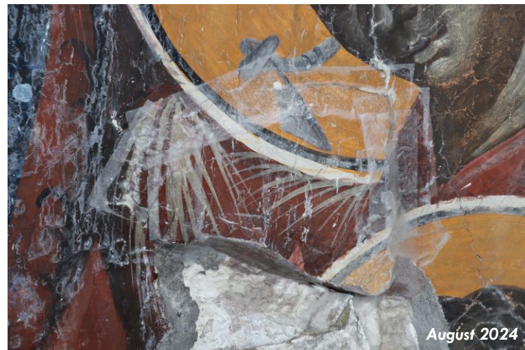
Images (Right and below): The Church of the Virgin, main space, south arm, vault level, west wall; Condition after temporary stabilisation.
