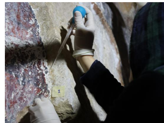
Above and right: Application of a "micro-injection solution" via pipette and testing different micro-injection materials
