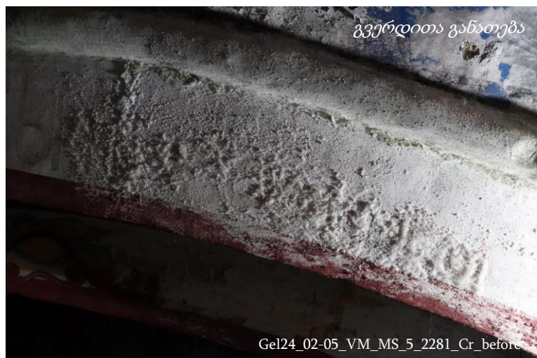
Above: Condition before salt removal
