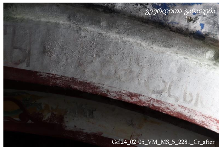
Above: Condition after salt removal
