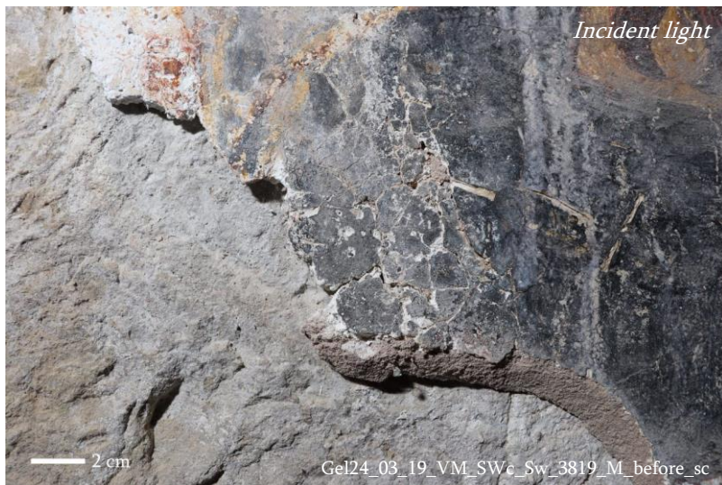
Above: Condition before intervention – loss of previous edge repair and original plaster. Plaster separation from stone support.
