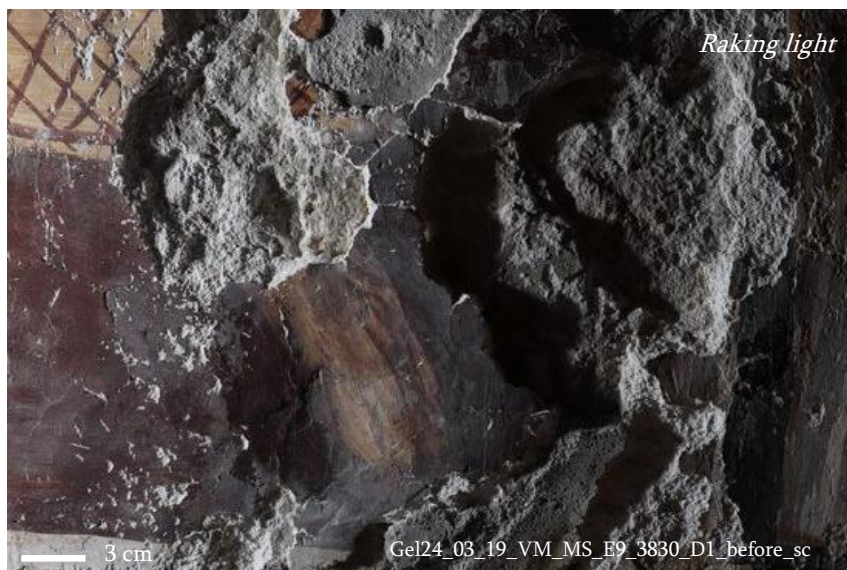
Above: plaster delaminated from stone support.
