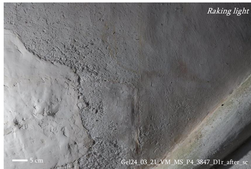
Above: Condition after salt removal
