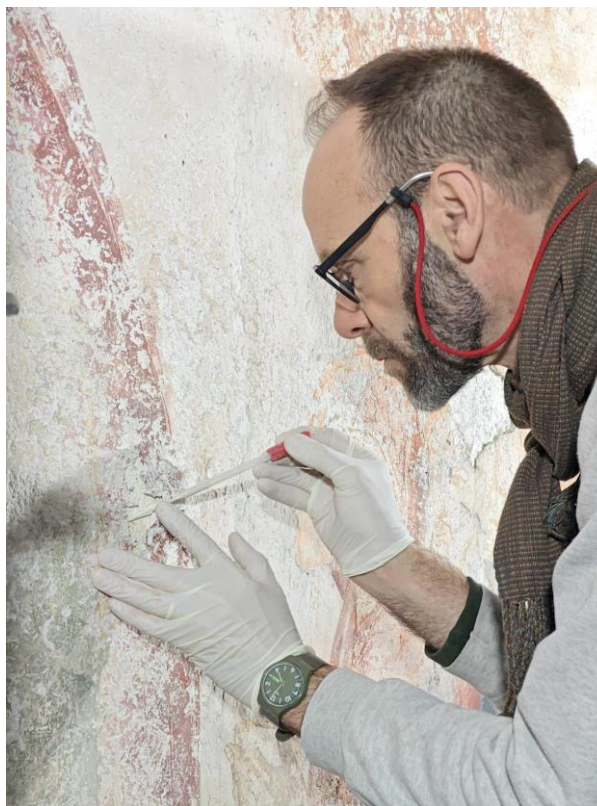
Above and right: Application of a "micro-injection solution" via pipette and testing different micro-injection materials
