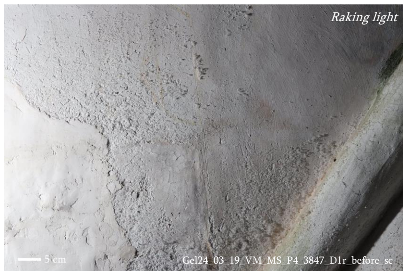
Above: Condition before salt removal
