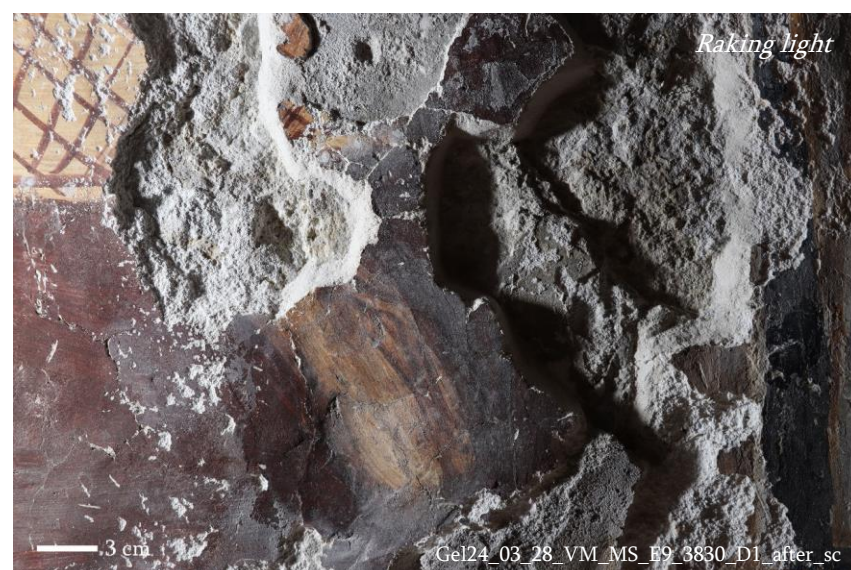
Above: plaster after re-adhesion and edge repair.
