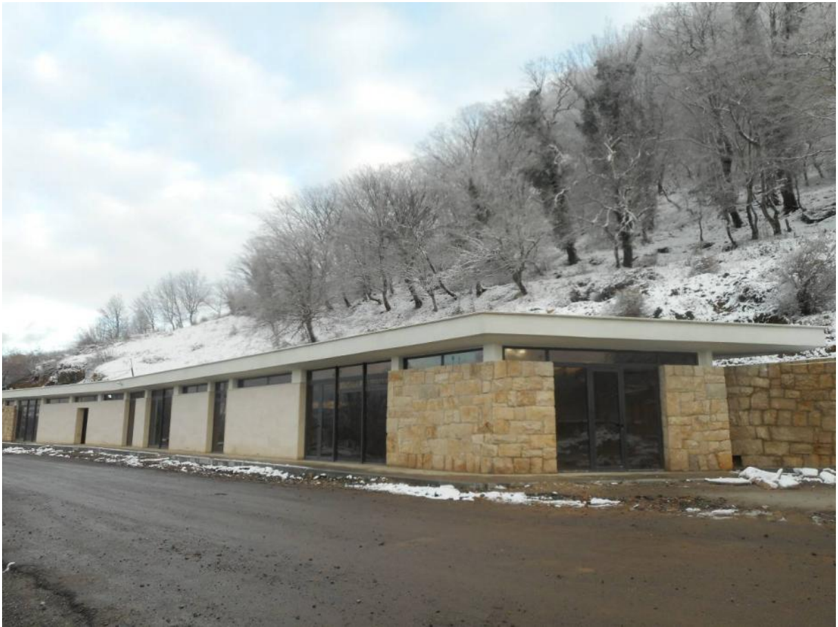
New visitor centre near the entrance of the Monastery (December 2016)
