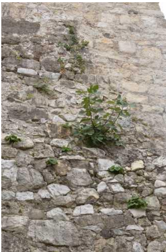
Shoots of fig tree on the west wall of the south gate
