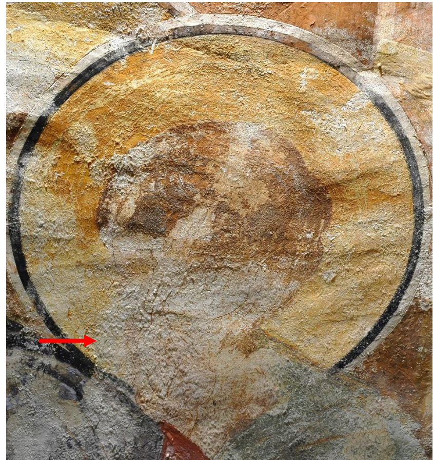
Condition today, Salt efflorescence July, 2023
