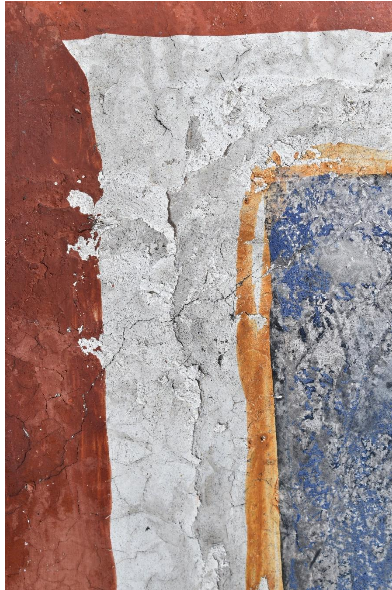
Plaster joint of the scene's frame
