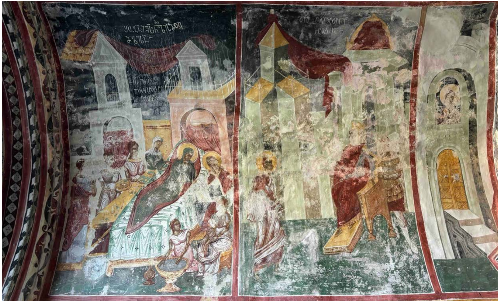
Above: The vault of the North Entrance showing effects of rainwater infiltration and transportation of damaging salts. This typifies inherent conditions in many parts of the Gelati complex
