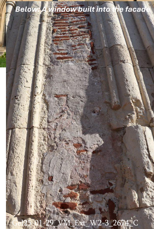
Below: The bricks and mortar used in the window.
