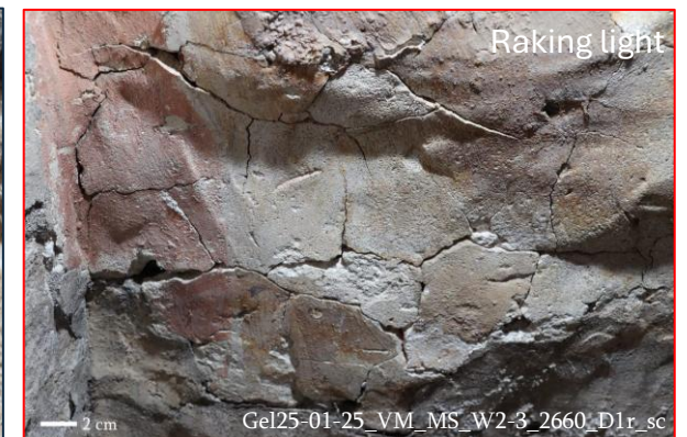
Above: Cracked and disintegrated paint, fragmentation and blistering of the paint. 14
