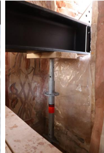
Above: Photos of the metal construction from the interior side. The openings from the facade side were temporarily covered with thick polyethylene film to prevent water ingress.
