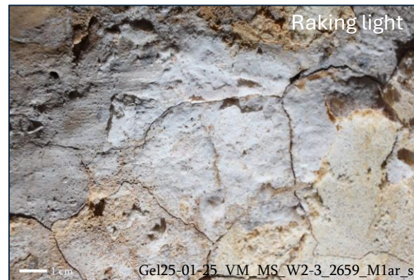
Above: Cracked and disintegrated paint, partial and complete disintegration of the paint. Crusty salt.
