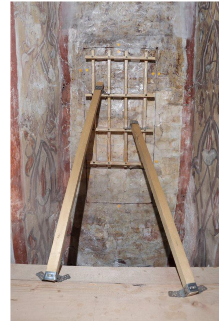
Left: Process of attaching the wooden frame to the treated painted surface.
