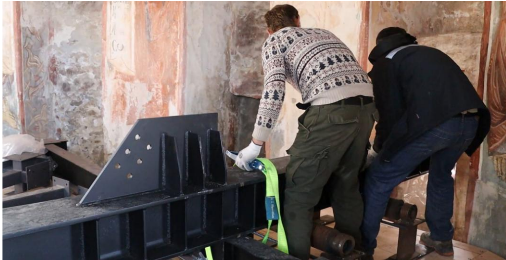
Above: The process of sliding into the opening using the metal construction rails.
