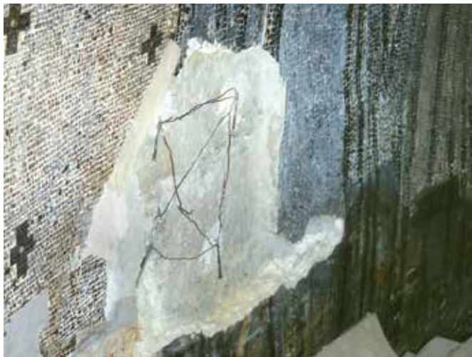
23. Metal wires introduced into the mosaic mortar setting during the restoration of the '80s
