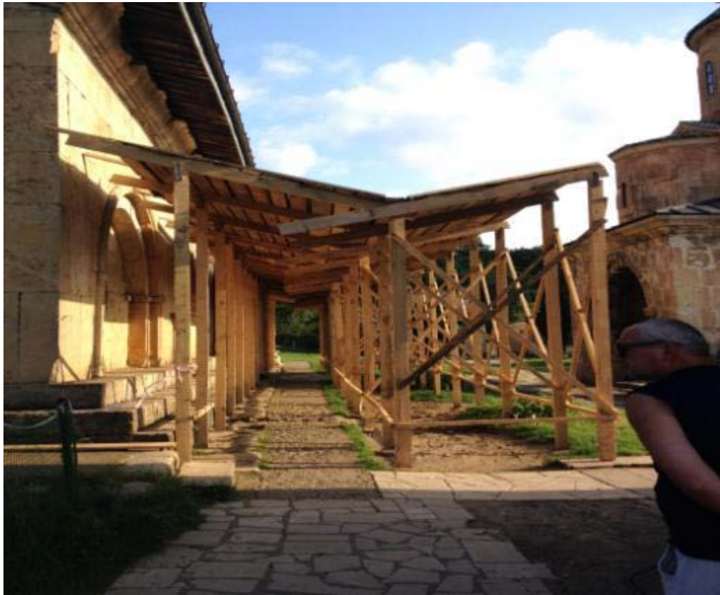
9-10. Construction of Scaffolding on the Western facade
