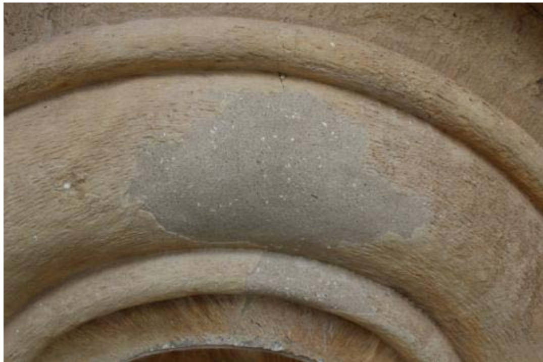
36-37. Consolidation of missed parts of masonry by lime and pozzolana, Drum Upper level
