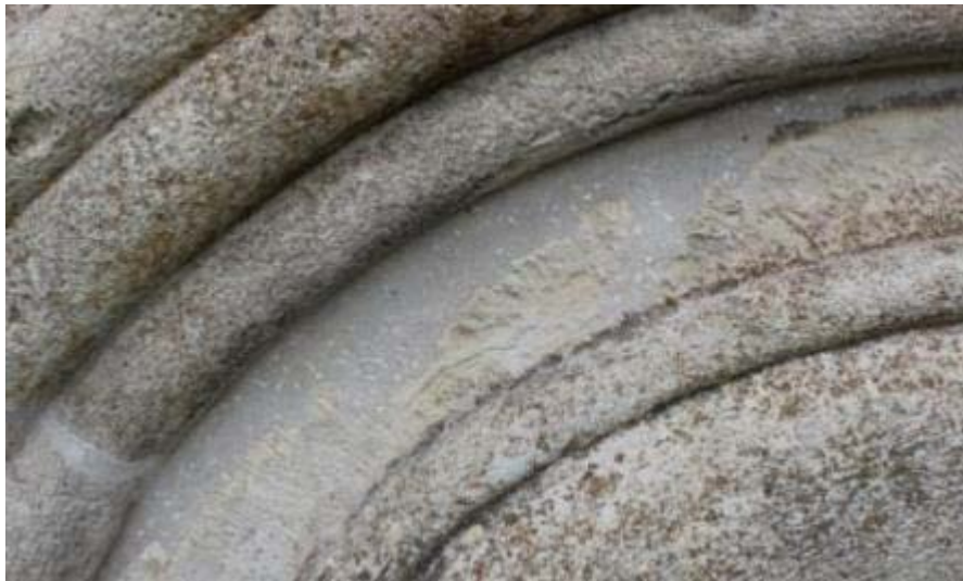
27-29. Filling of Joints, Drum Upper level, Uppers side of the window, Southern side
