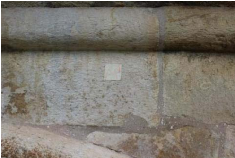
30-31. Filling of Joints, Drum Upper level, Northern side
