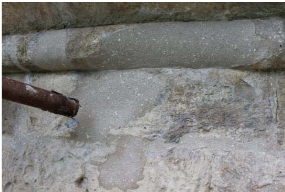
32-33. Filling of Joints & Consolidation of missed parts of masonry by lime and pozzolana, Drum Upper level, North-Western side
