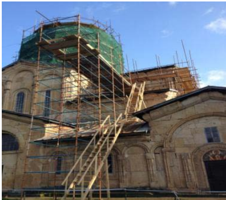
11-12. Construction of Scaffolding on the Northern facade
