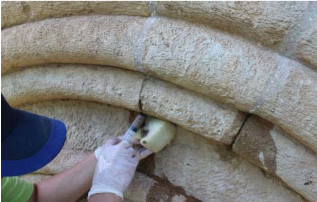
19-20. Injection with lime solution
