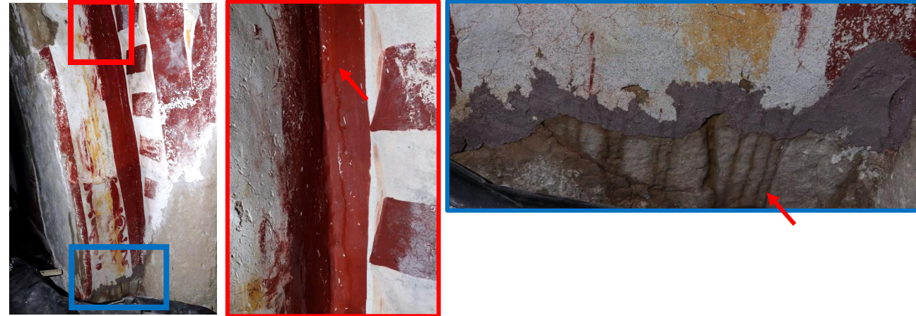
On the left: Main space, vault of the west arm, northern part of arch. Evidence of the liquid water flow
