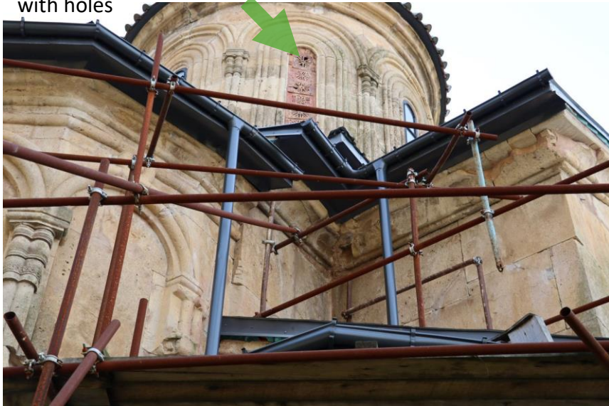
St. George,, dome north-east window made of ceramic tiles with holes
