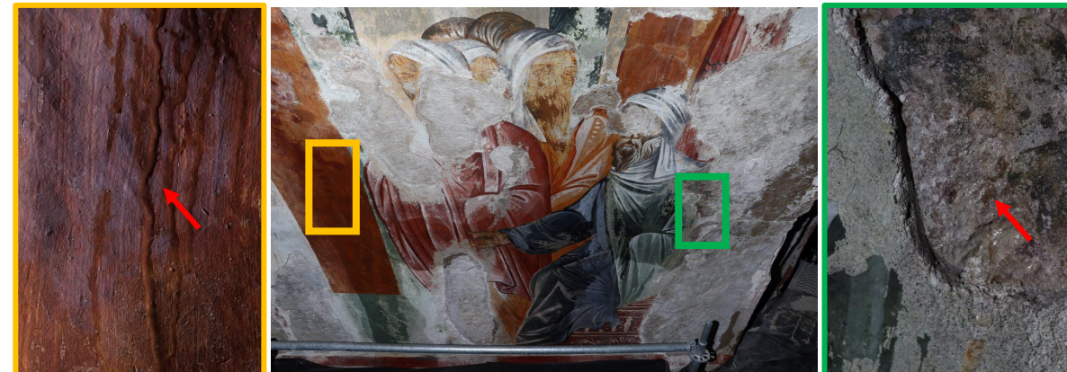
On the left: Main space, vault of the west arm, northern wall, scene N6. Evidence of the liquid water flow on the two spots (see red arrows)
