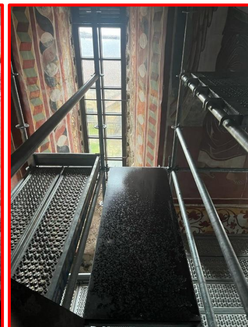
Wet part of the scaffolding. Water was splashed through window shutter.
