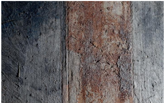
Compositional layout on wet plaster, snap-line. 2025
