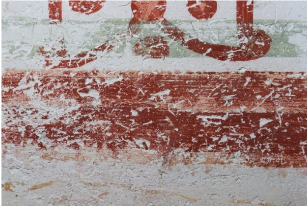
Compositional layout on wet plaster, pigmented snap-line. 2025
