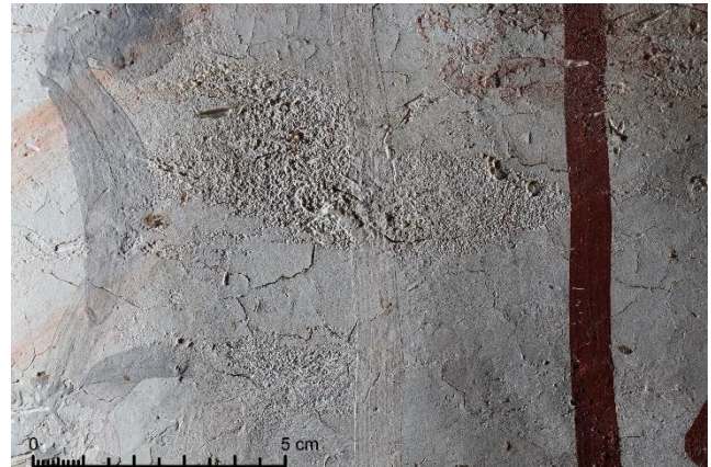
Probable wooden tool traces on plaster surface. 2025
