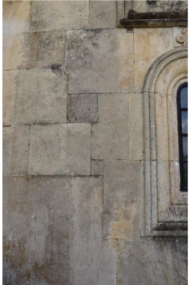
South façade showing small incorporated stones in the facing masonry. 2025
