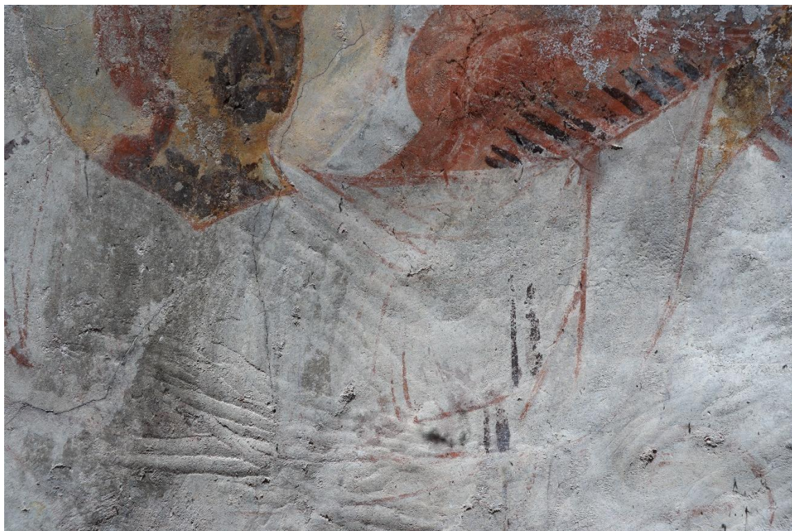
Plaster finishing traces, vault. 2025
