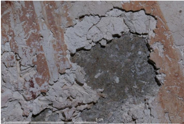
Plant fiber in both plaster layers. 2025
