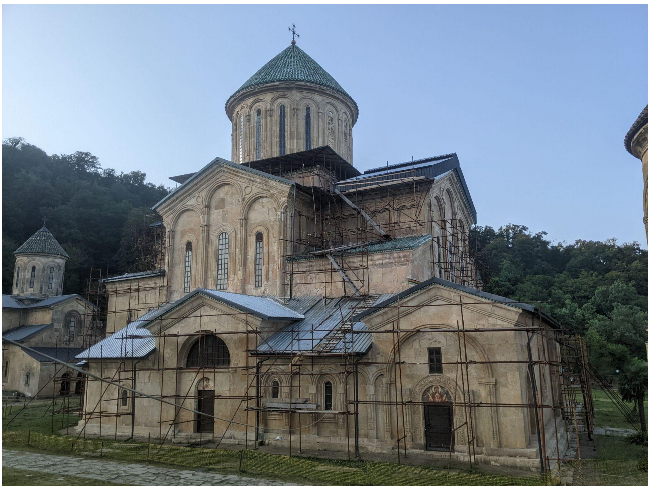
Figure 13. The WA temporary covering, global view (photo by Architect Lasha Shartava).
