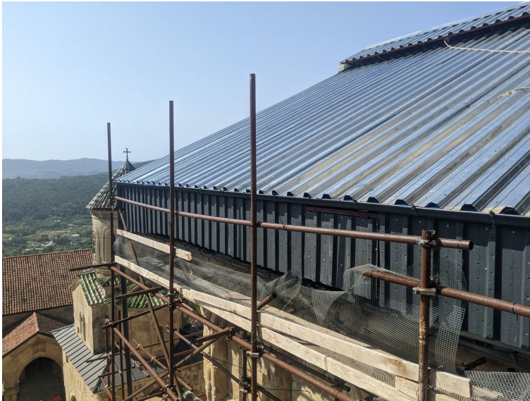
Figure 9. The WA temporary covering, view from the outside (photo by Architect Lasha Shartava).
