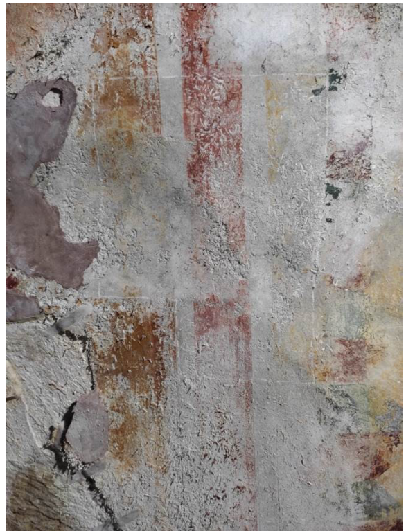
Consolidation plaster (intonachino) with Ammonium Oxalate
