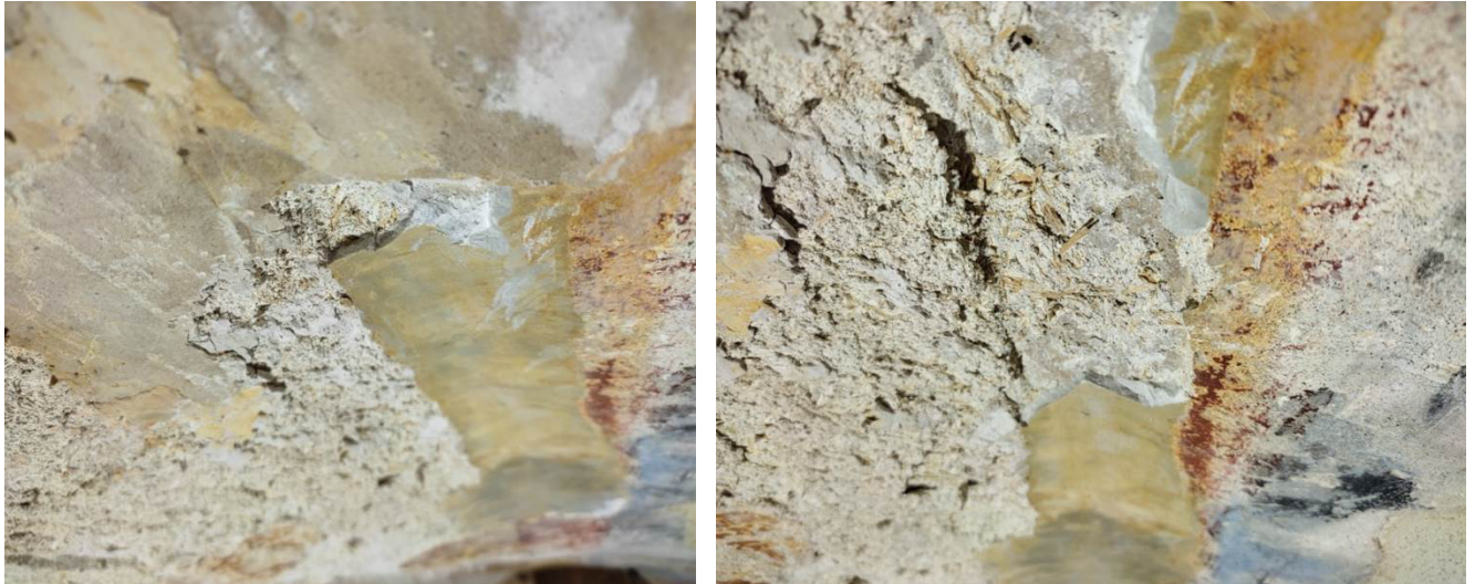
Removing the old stucco fillings around the vault cross
