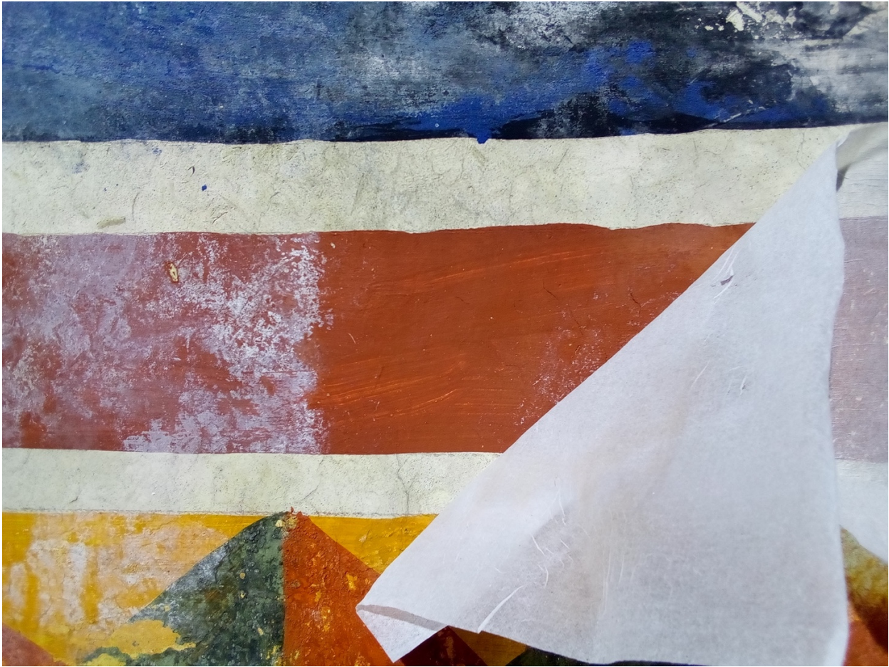
North wall - Carbonation cleaning
