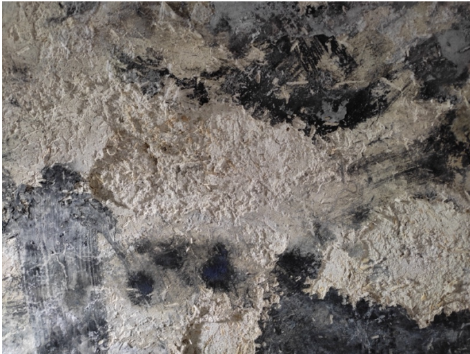
Disintegrated plaster (intonachino) consolidation
