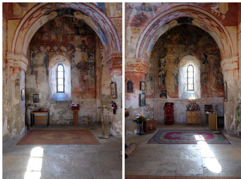
Figures 22 and 23 - Views of the interior spaces of St. George with widespread damage to the paintings which are lost, for the most part, in the lower part (from MCT SG report).
