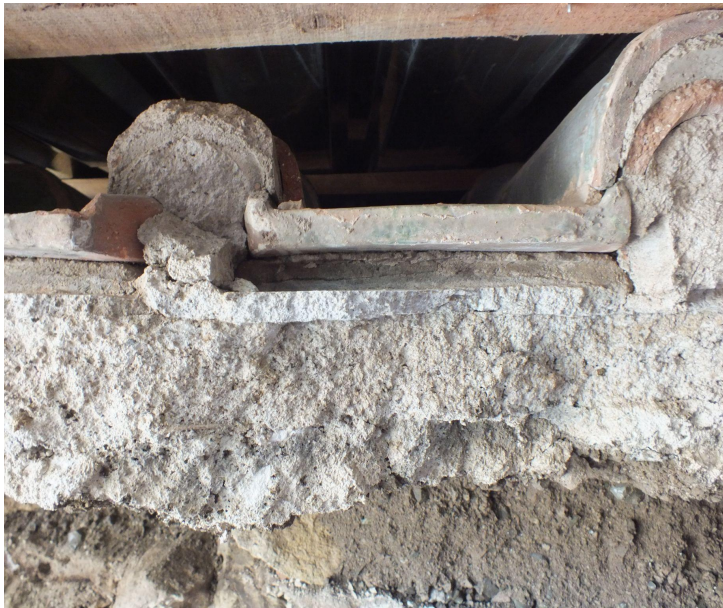
Figure 2 - Thick layer of mortar insert during the last intervention. It is possible to see that in this pitch (belonging to the West Arm) there is no insulation layer;
