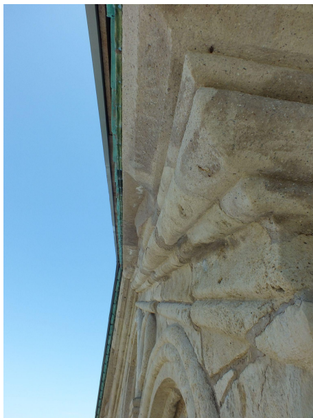
Figure 8 - Insufficient overhang of the roof in the West Arm facade.
