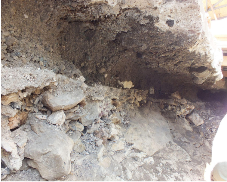
Figure 6 - Roof stratigraphy: it is possible to see the wet filling under the mortar layer.
