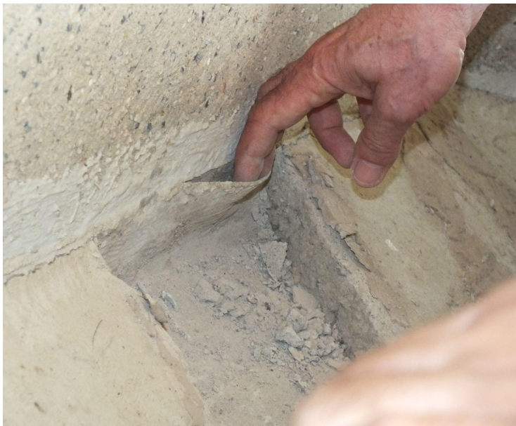
Figure 4 - Connection between the insulation layer and the vertical wall: the insulation is tucked up by just a few centimetres, insufficient for effective insulation.
