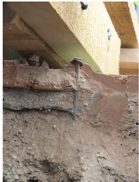
Figure 4 - Connection between the insulation layer and the vertical wall: the insulation is tucked up by just a few centimetres, insufficient for effective insulation.
