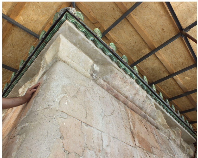
Figure 8 - Insufficient overhang of the roof in the West Arm facade.
