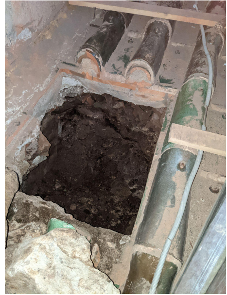
Figure 6 - Roof stratigraphy: it is possible to see the wet filling under the mortar layer.
