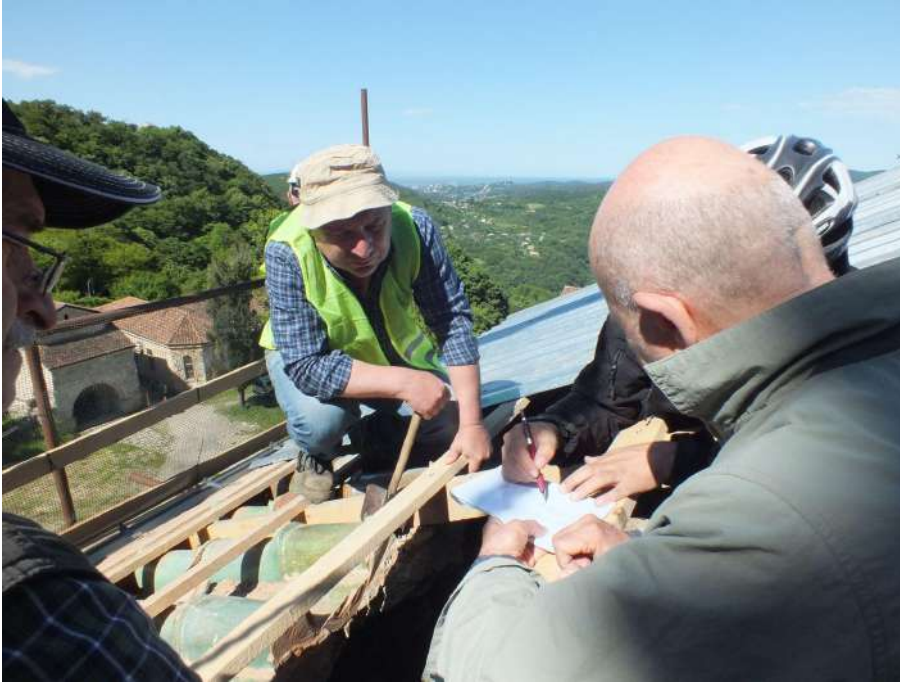
Southern wall of West Arm. Discussion about the crack and the materials found in the filling of the under roof.
