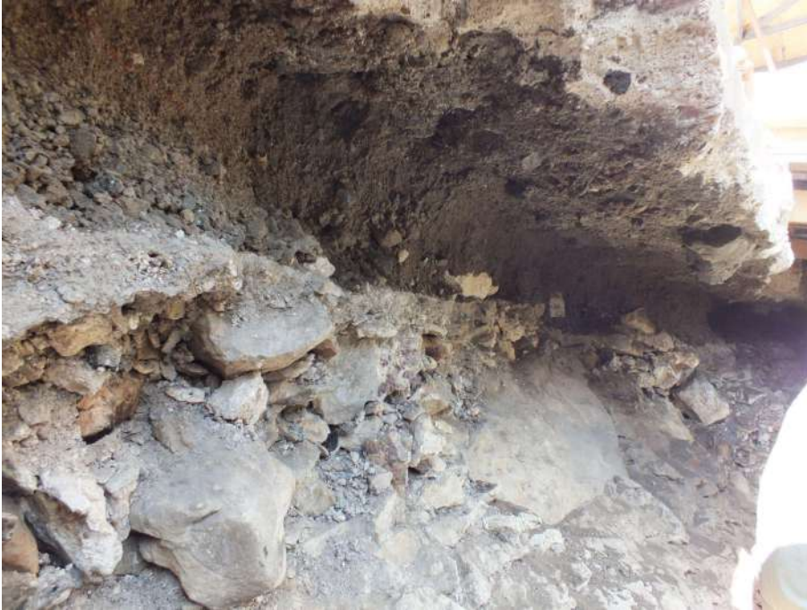
Southern wall of West Arm. Different layers of the under-roof filling.
