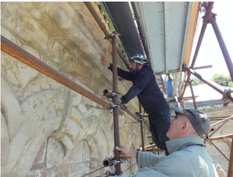
Southern wall of West Arm. Inspection of the external facade.
