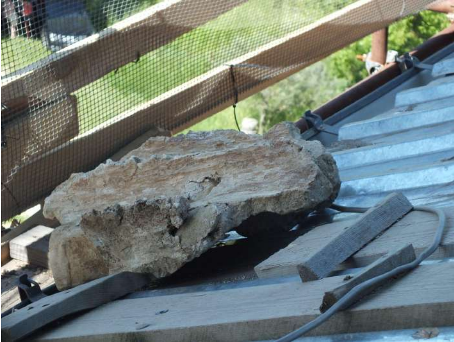
Ancient mortar filling with the imprint of timber.
