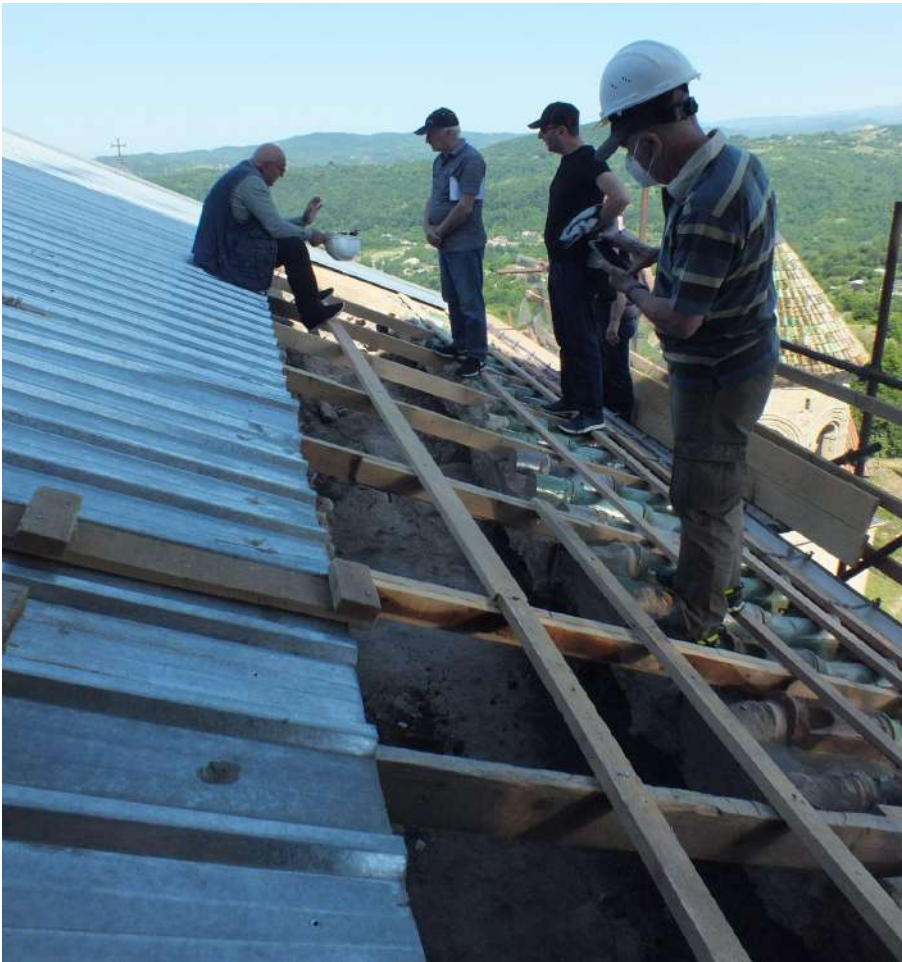
Northern wall of West Arm. Inspection with Eng. Zurab Okroshidze.
