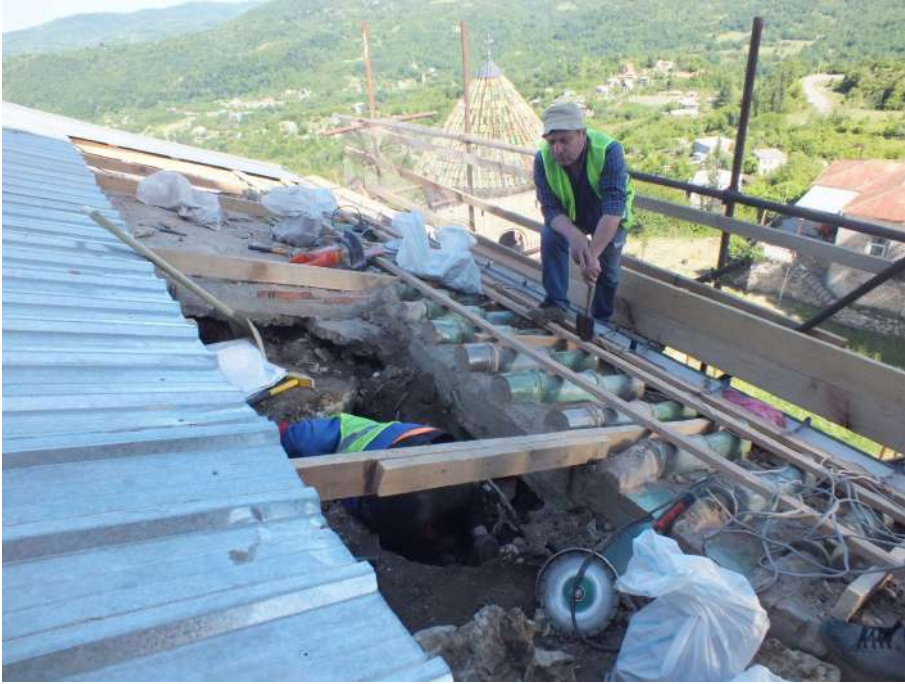
Northern wall of West Arm. Roof opening operations.
