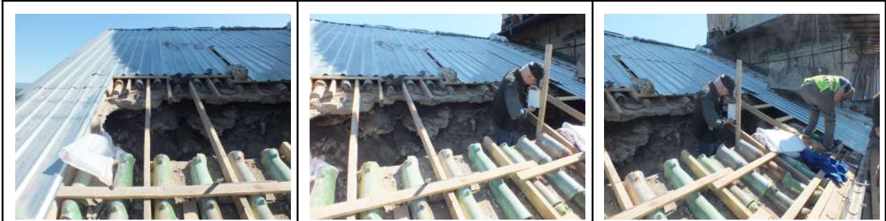
Southern wall of West Arm. The opening.
