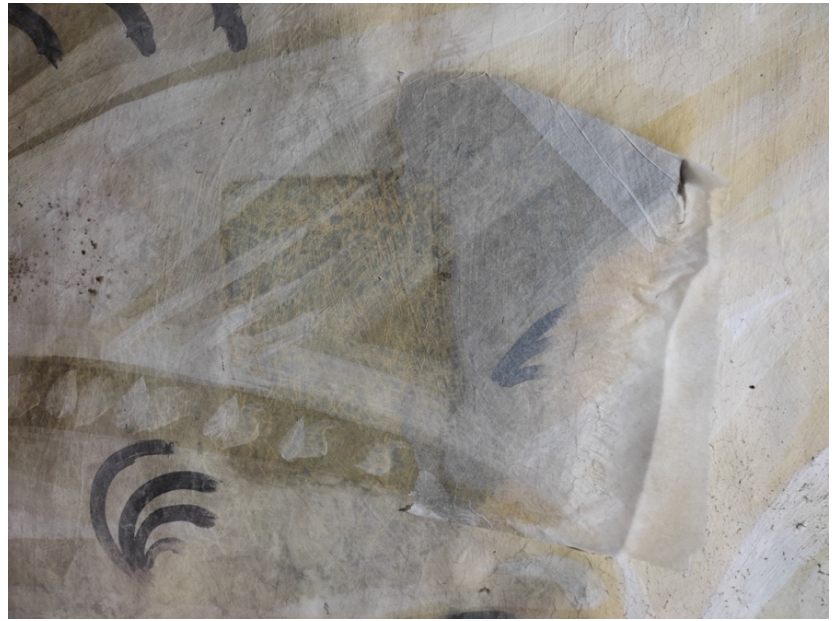
During the cleaning test
