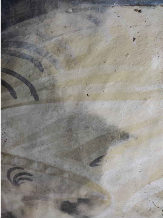
Landscape of the hill before cleaning: note the clear transition between the dirty and the light area that already looks clean
