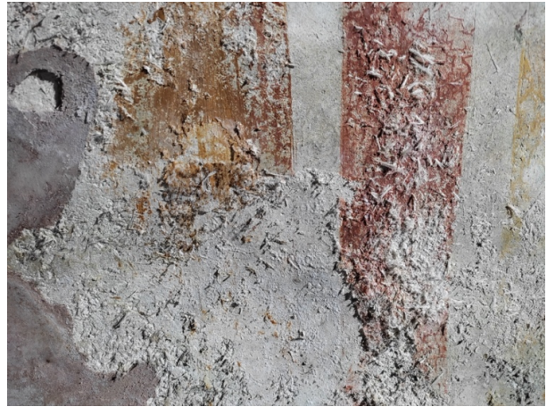
color disintegration by attack of salt crystals
