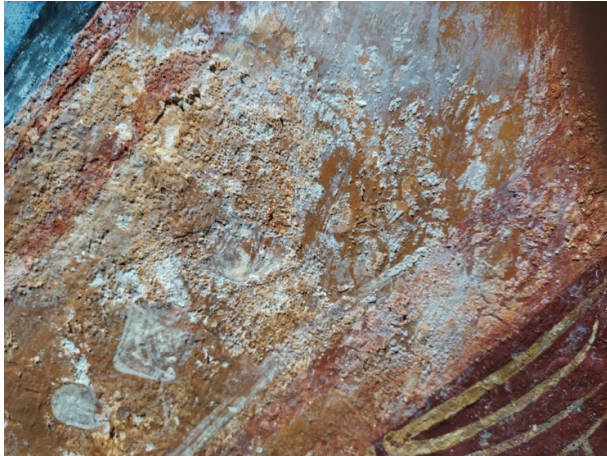
color disintegration by attack of salt crystals
