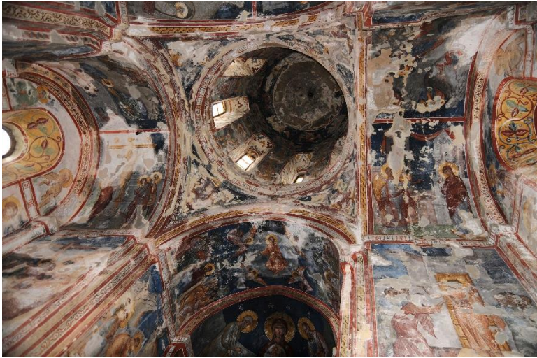
Fig. 60. Interior view to the cupola
