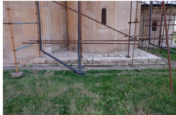
Figure 11: detail view of downpipes d10 and d11 with the manhole sm-5
