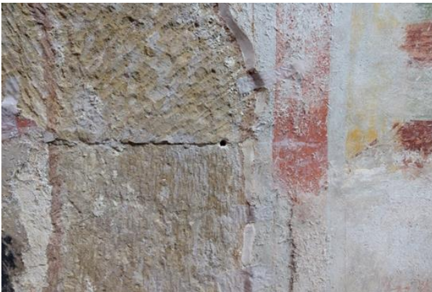
Figure 38: Point D, west wing vault, south side
