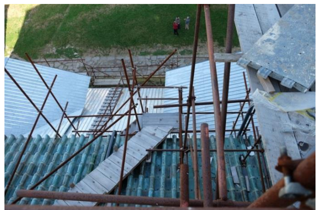
Figure 19: roof of the northern aisle, without temporary covers
