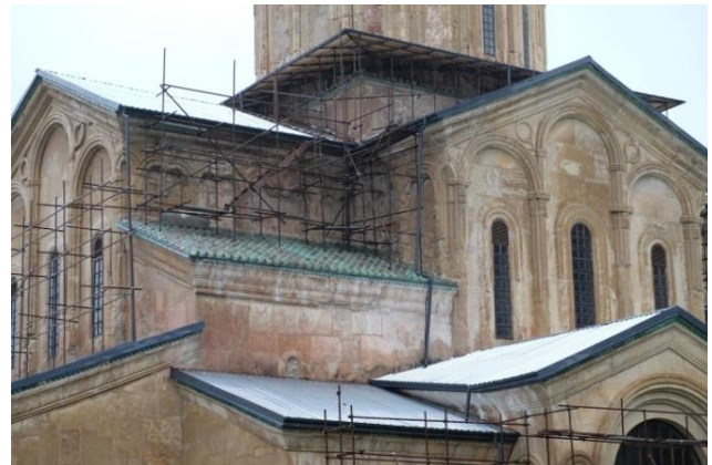
Figure 17: roof of the southern aisle, without temporary covers
