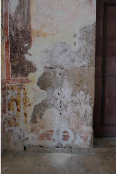
Figure 35: Point A, environment 2, on the side of the north entrance
