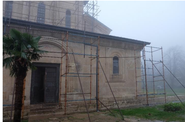
Figure 5: view of downpipes d2 and d3 in operation during the thunderstorm
