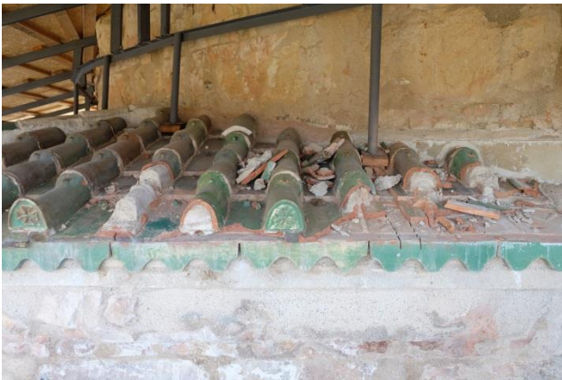
Figure 20: structure of temporary roofing shelter, elevated on roofing tiles layer
