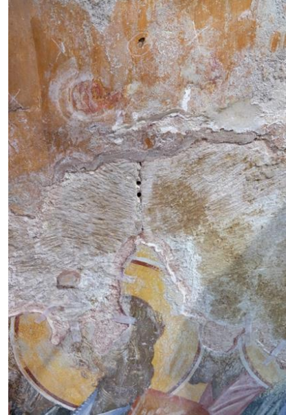
Figure 37: Point C, west wing vault, south side
