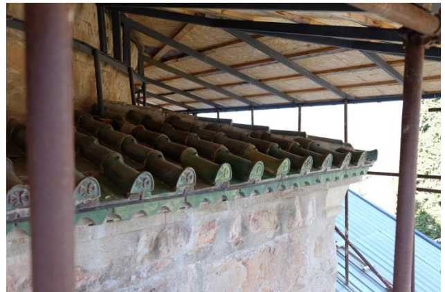
Figure 21: structure of temporary roofing shelter, elevated on roofing tiles layer
