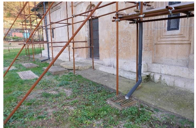
Figure 8: detail view of downpipe d15 with manhole sm-9
