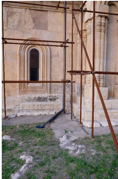
Figure 14: view of downpipe d4 with the manhole sm-1
