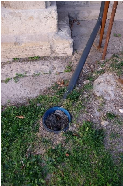
Figure 13: detail view of downpipe d5 with the manhole sm-5
