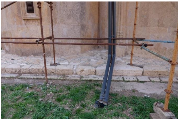
Figure 10: detail view of downpipes d8 and d9 with the manhole sm-4
