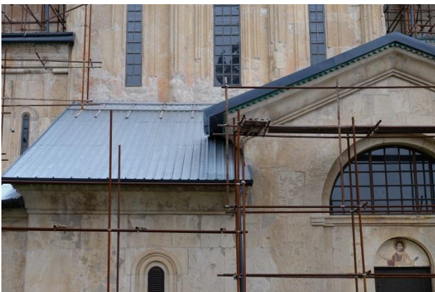
Figure 22: temporary roofing leaning against roofing tiles layer
