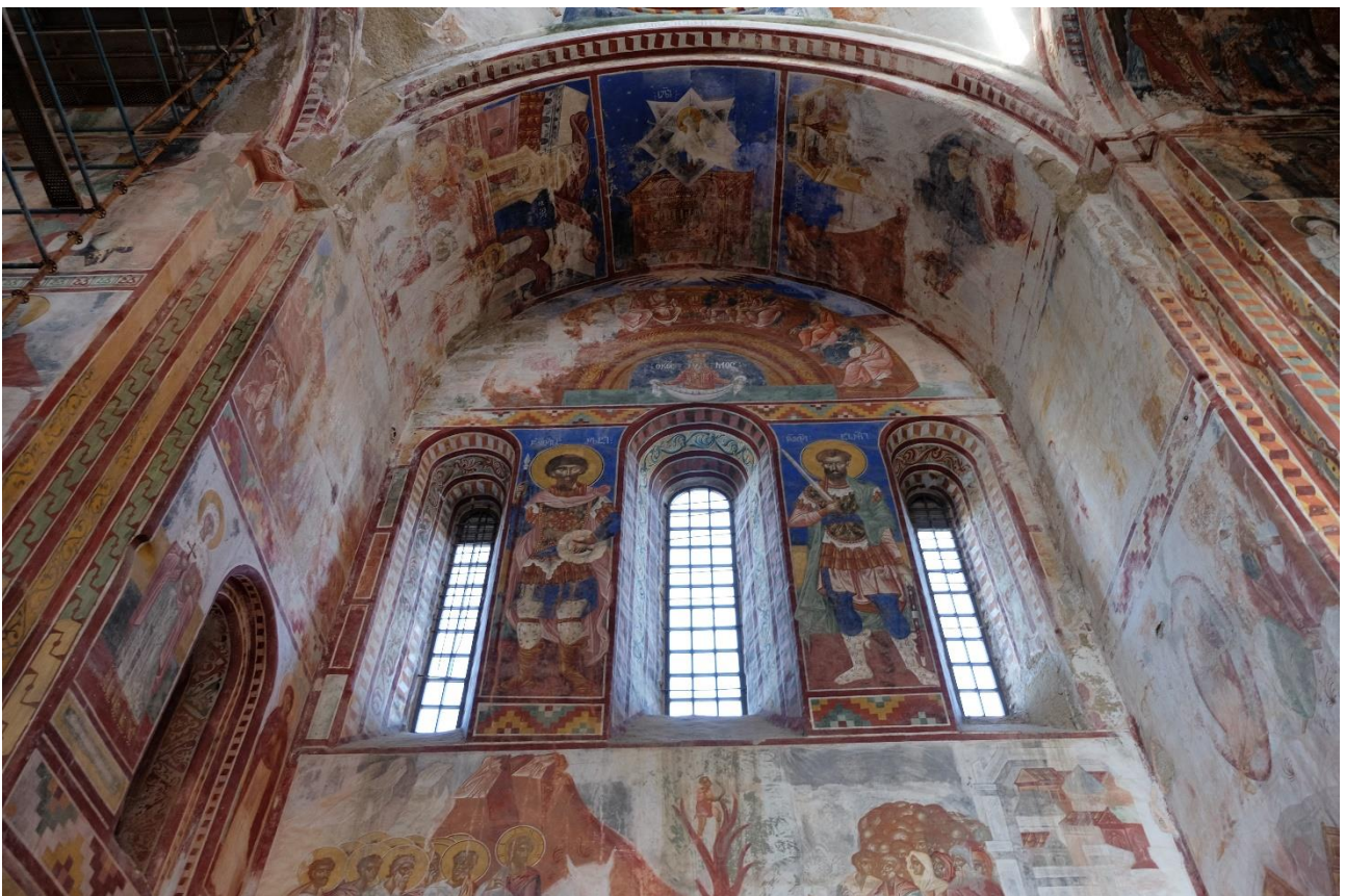
Figure 24: view of three windows overlooking the transept: the middle one only glazed, while equipped with 'anti-animal' net and a protective external shutter the side ones
