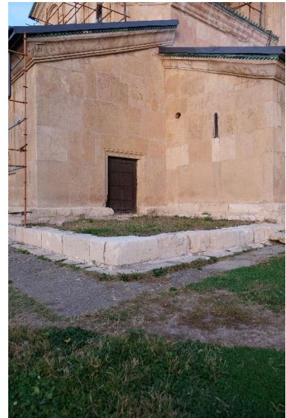
Figure 15: view of the south-west corner of the church
