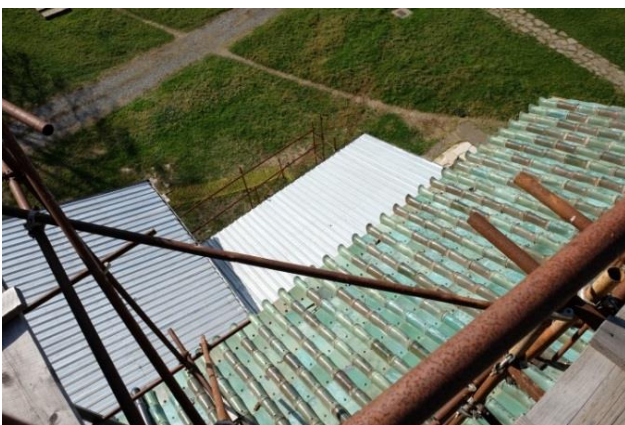
Figure 18: roof of the southern aisle, without temporary covers
