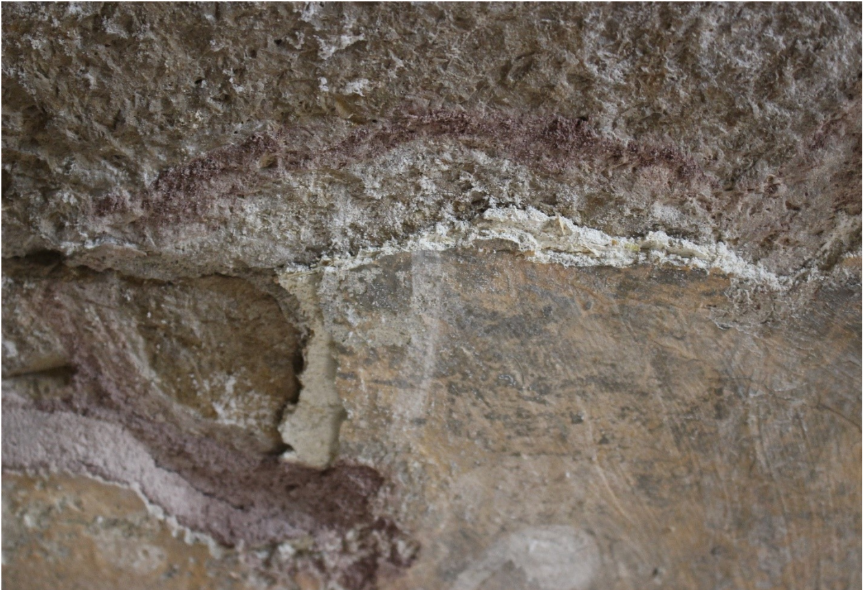
Detachment of portions of plaster due to the failure of the protections (tissues and stucco curbs)
