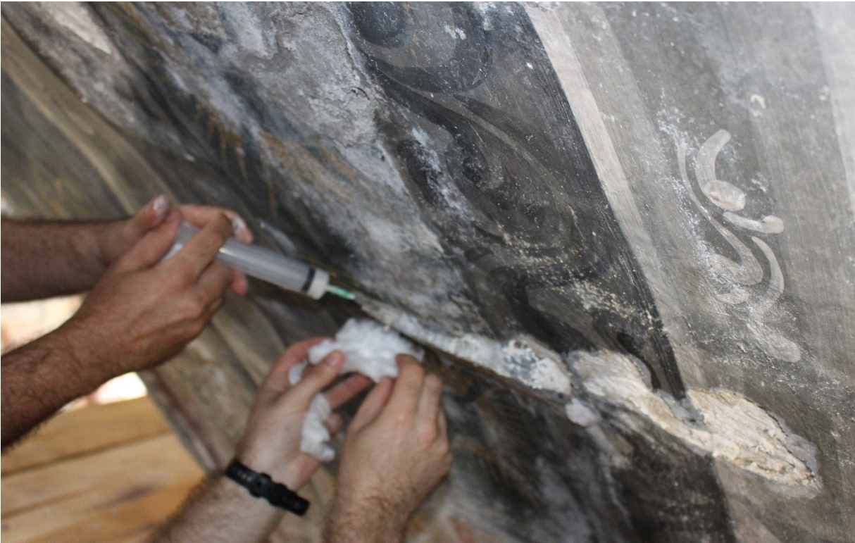
Consolidation of plaster detachments
