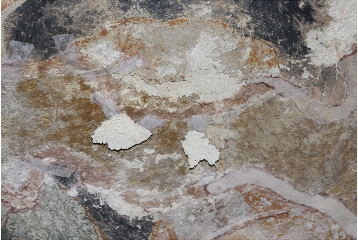
Detachment of portions of plaster due to the failure of the protections (tissues and stucco curbs)
