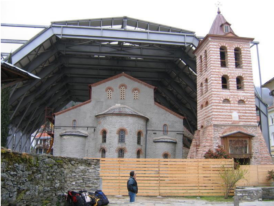
Fig.4. Protaton Church – The protective metal scaffolding.
