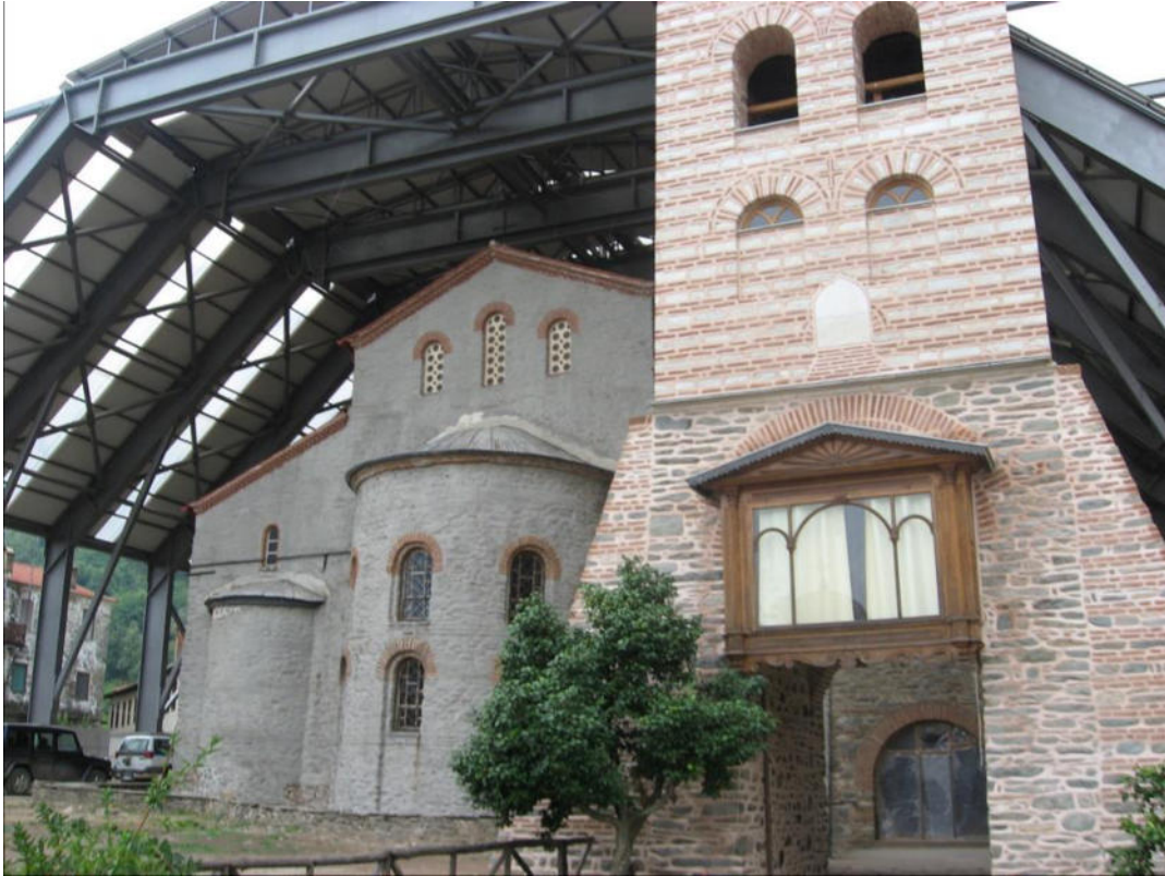
Fig.5. Protaton Church – The protective metal scaffolding.
