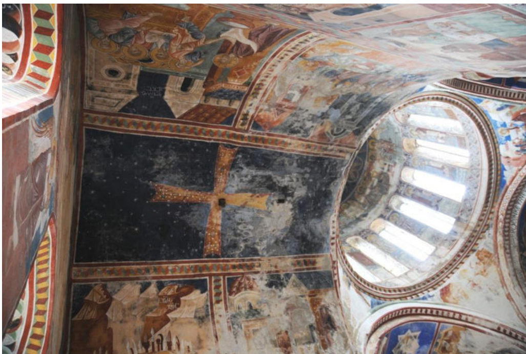
Church of the Virgin: Barrel-vaulted western cross arm (from the Report of the joint World Heritage Centre /ICOMOS/ICCROM Advisory Mission to Bagrati cathedral and Gelati monastery, March 2010)
