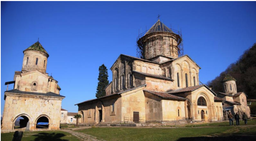
The monastery complex in 2015.
