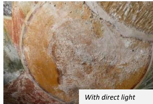
Condition as per April 30, 2020, before partial removal of salt
