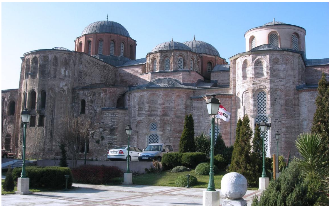
Fig. 46. The Church of Christ Pantokrator, the Imperial Chapel and the Church of the Theotokos Eleousa in the Pantokrator Monastery, Constantinople
