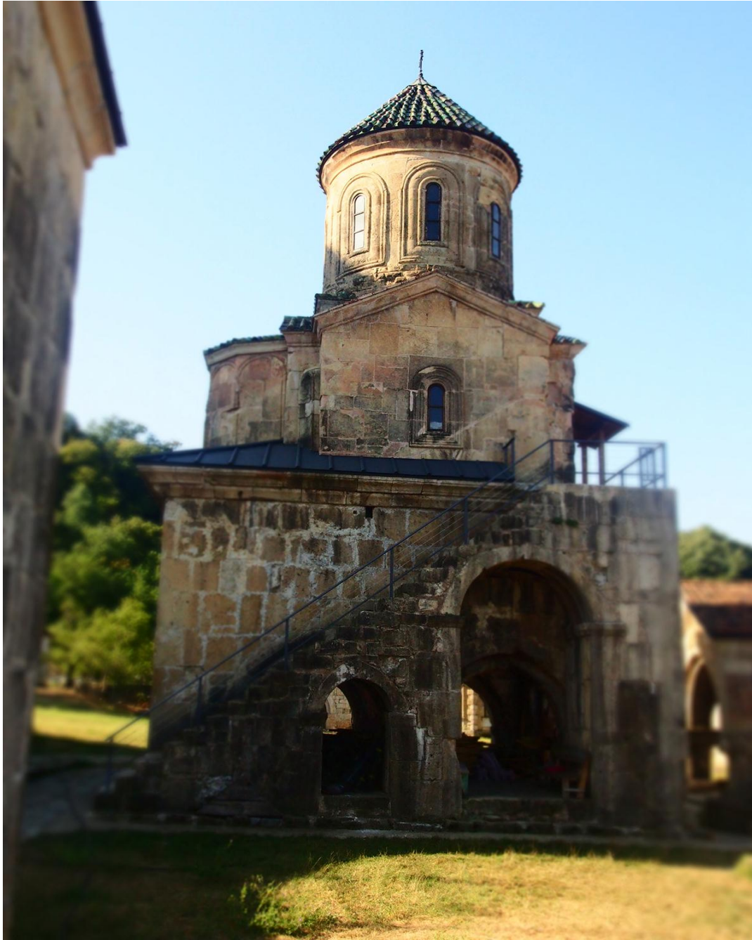
Fig. 22. Church of St Nicholas seen from the north-east (photo ST.)
