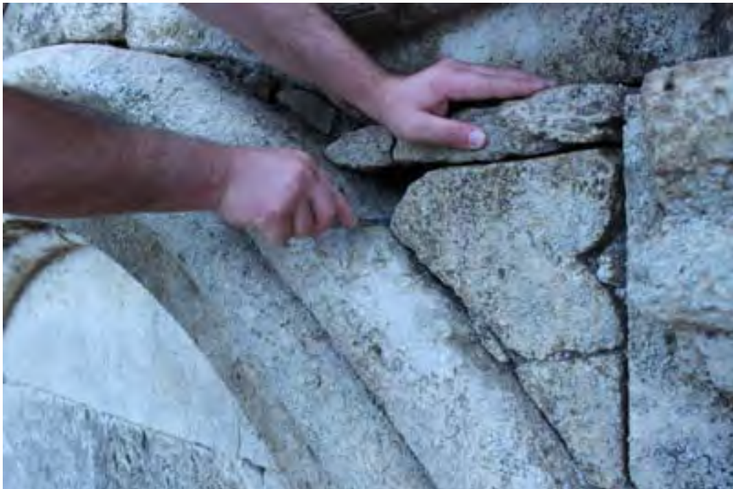
North façade of the Church of the Virgin at Gelati Monastery
