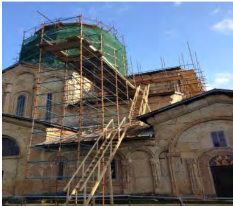
11-12. Construction of Scaffolding on the Northern facade
