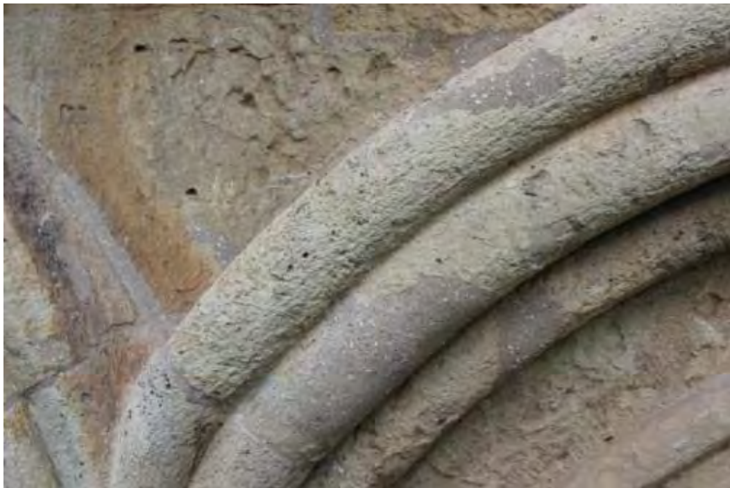
40-41. Consolidation of missed parts of masonry by lime and pozzolana. Northern side
