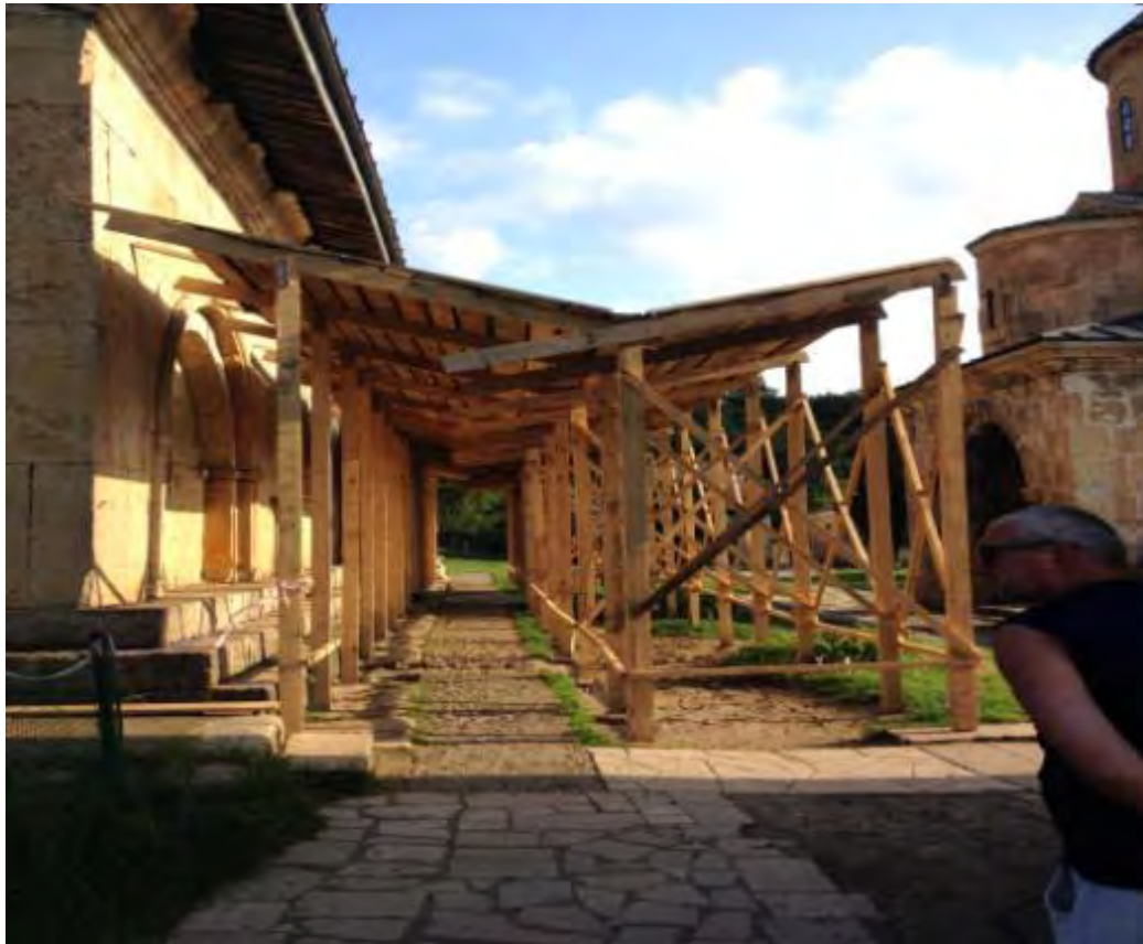
9-10. Construction of Scaffolding on the Western facade
