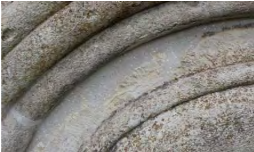
27-29. Filling of Joints, Drum Upper level, Uppers side of the window, Southern side
