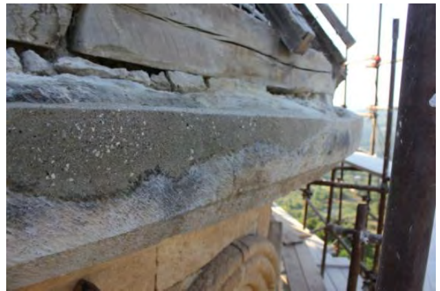
Fig. The cornice detail after the reconstruction
