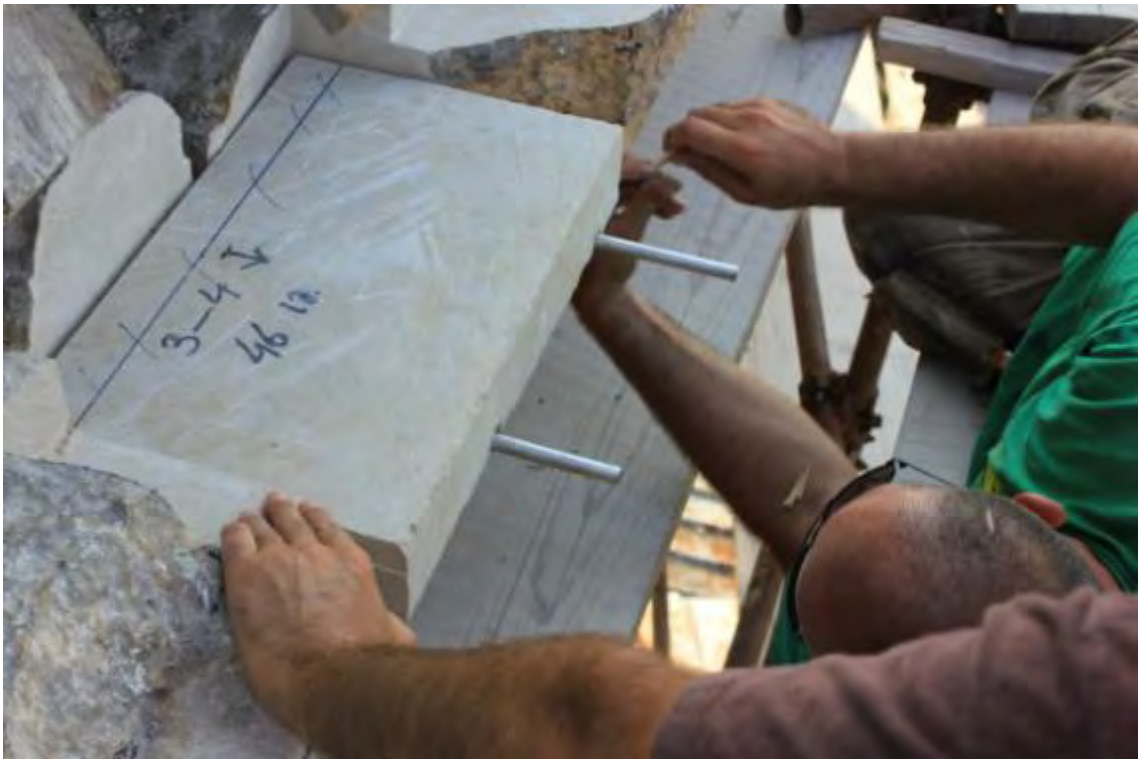
Fig. Fixing the stone
