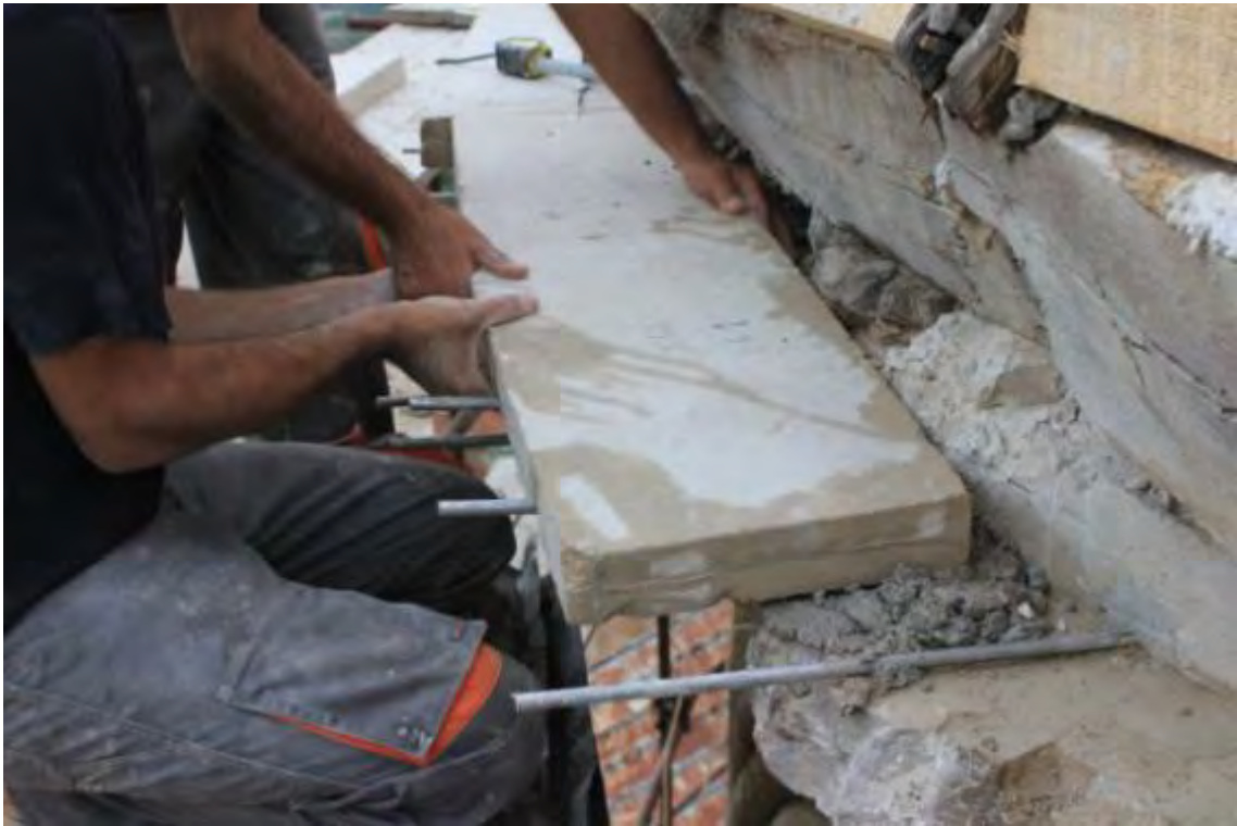
Fig. Fixing with the lime mortar
