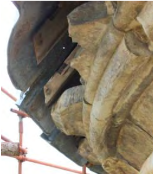
Fig. Rafters before the shortening
