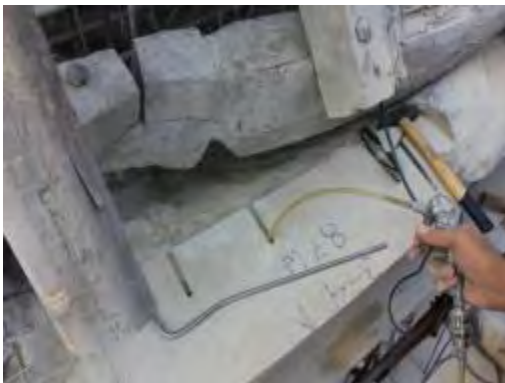
Fig. Cleaning anchoring holes
