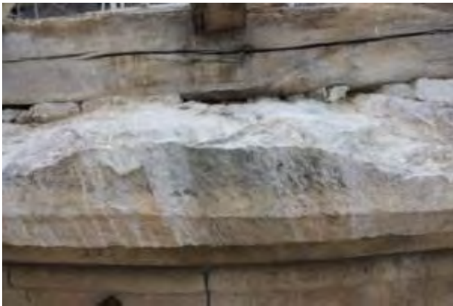
Fig. The cornice stone before the reconstruction
