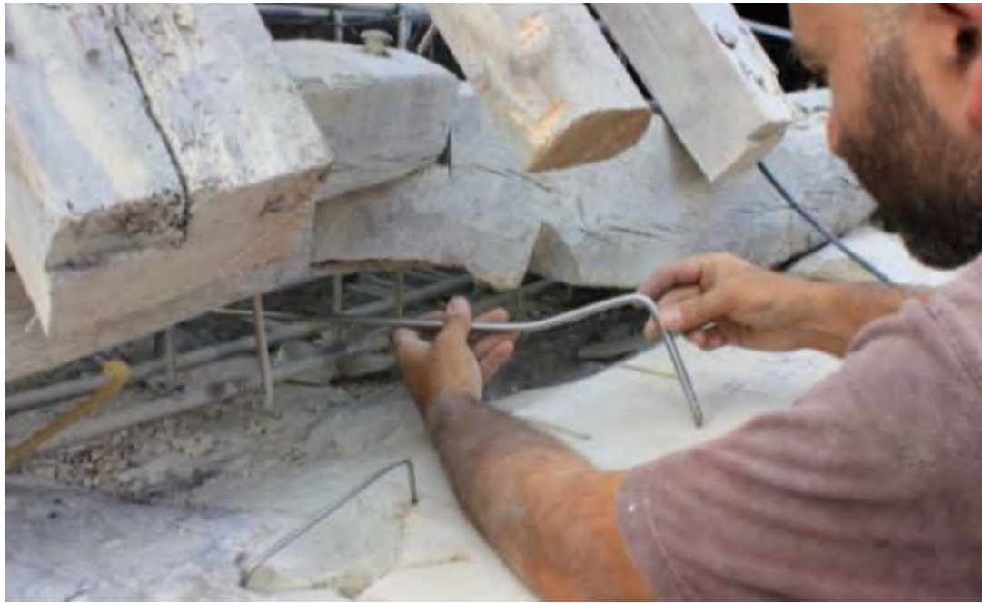
Fig. Anchoring
