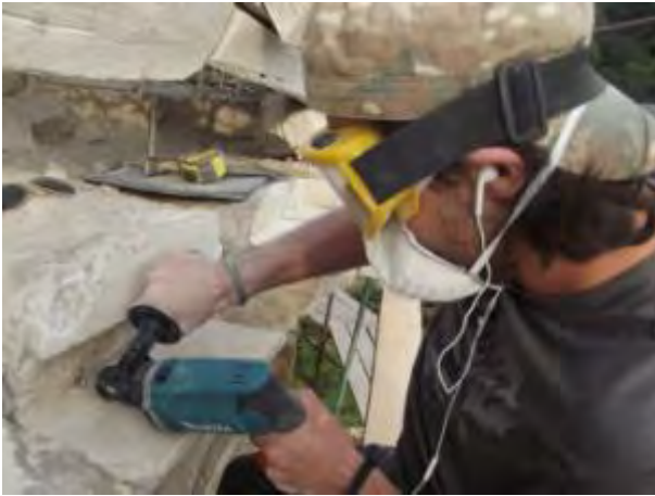
Fig. Preparing the holes for anchoring
