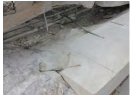
Fig. Anchored stone details
