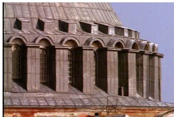
Figures 9, 10. St Sophia in Constantinople – reinforcement of the piers between the windows, after the collapse of the original dome in 559
