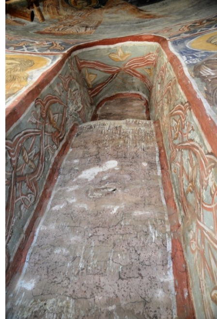
Figure 8. Walled drum window openings
