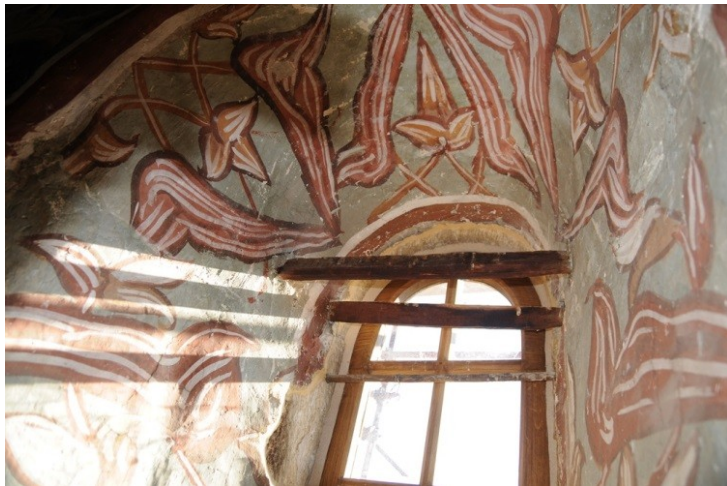
Figure 7. Wood tie-beams still preserved on drum window openings
