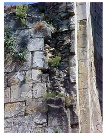
6. The condition of walls before consolidation
