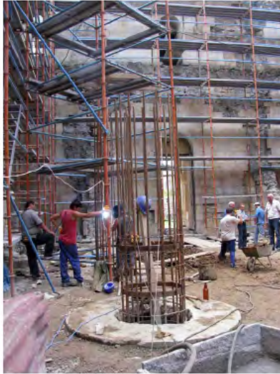
Current reconstruction works
