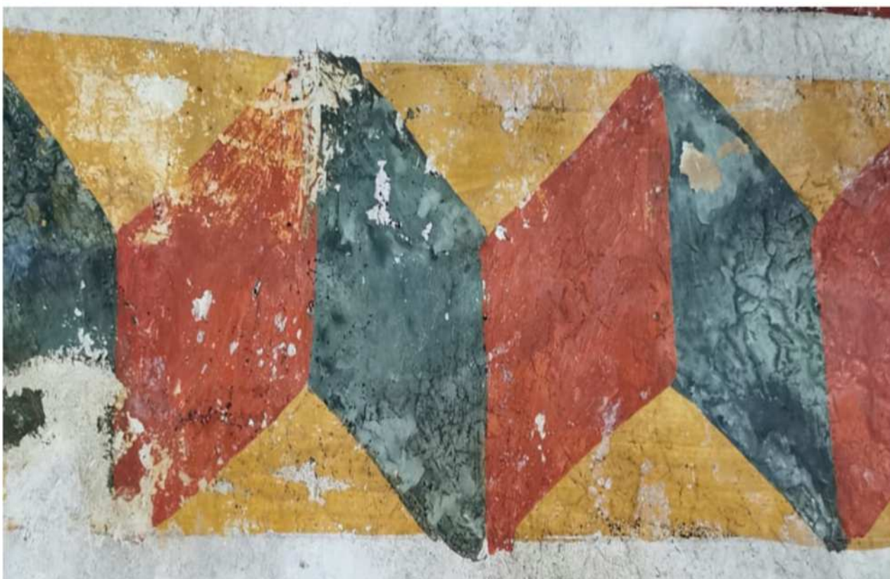
Fixing of the paint film and removal of saline efflorescence
