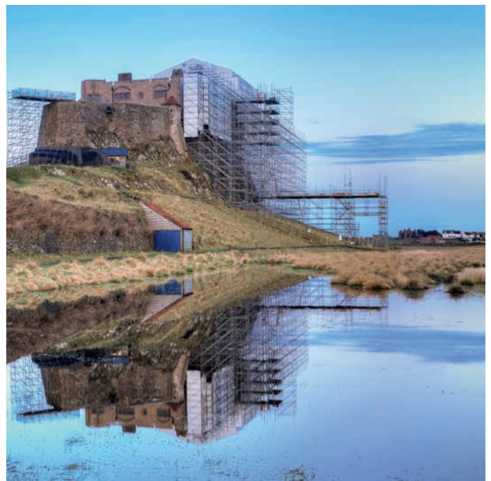
Example of support scaffolding for a free-standing facade
