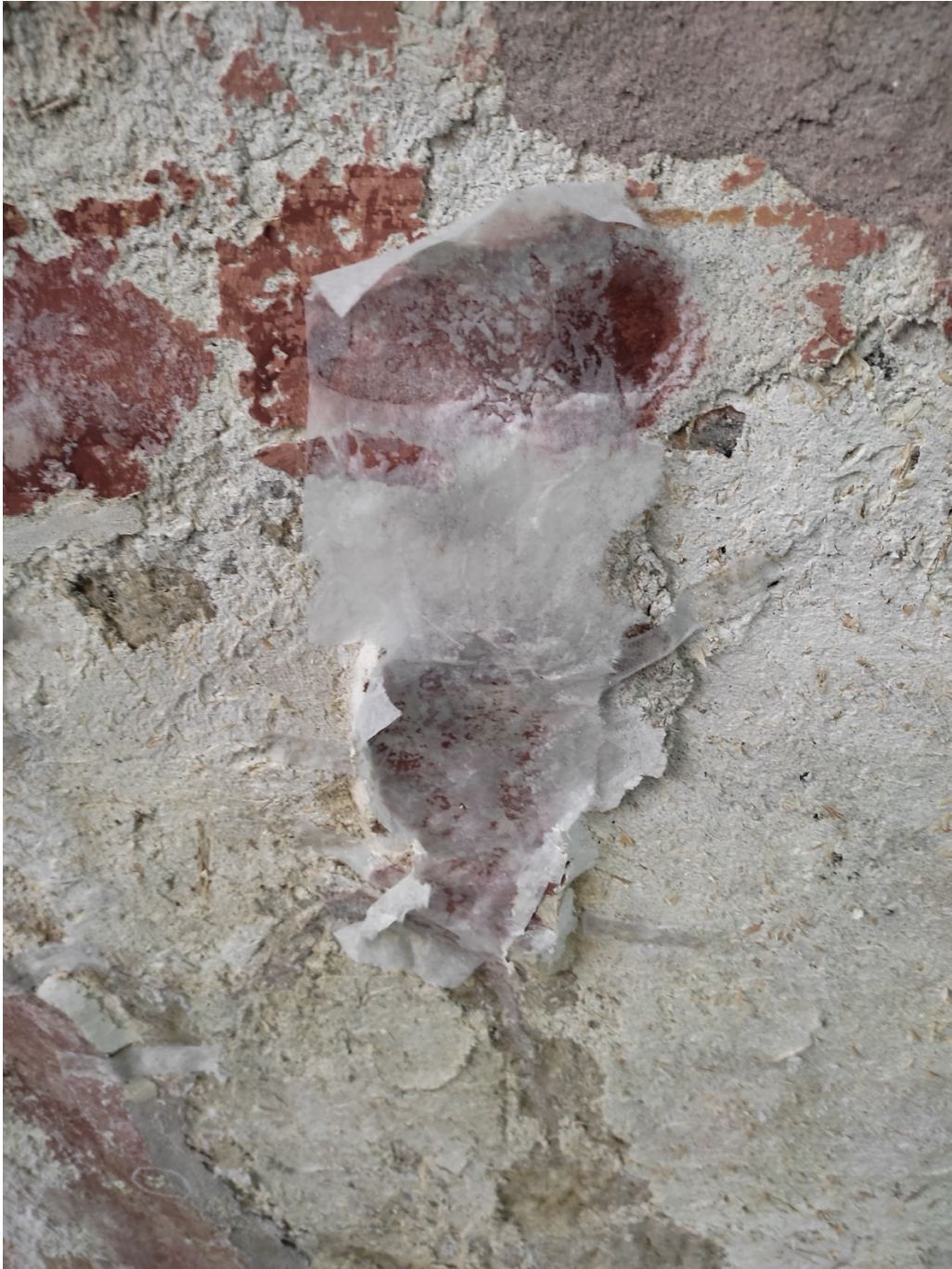
application of velinatura with Paraloid B72 to consolidate the plaster
