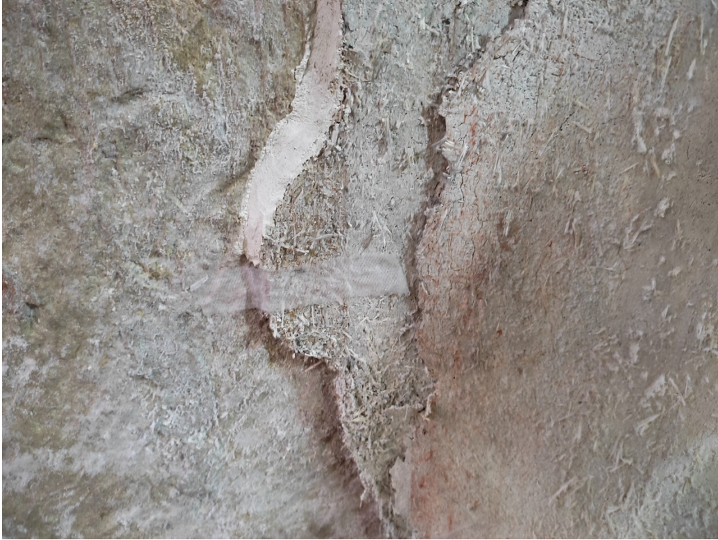
temporary anchoring grouting for consolidation of plaster
