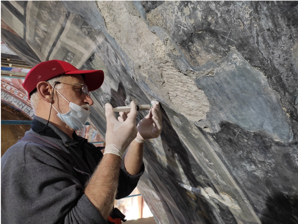
Georgian Conservator while consolidating the plaster
