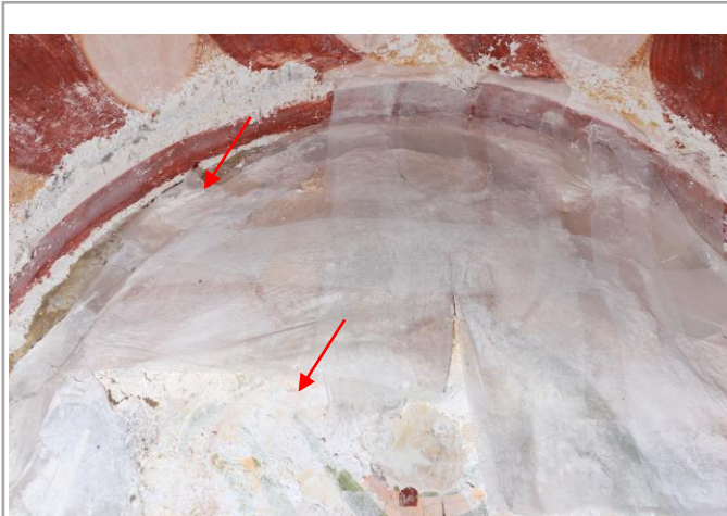
Two months after reinforcement. May 2024
