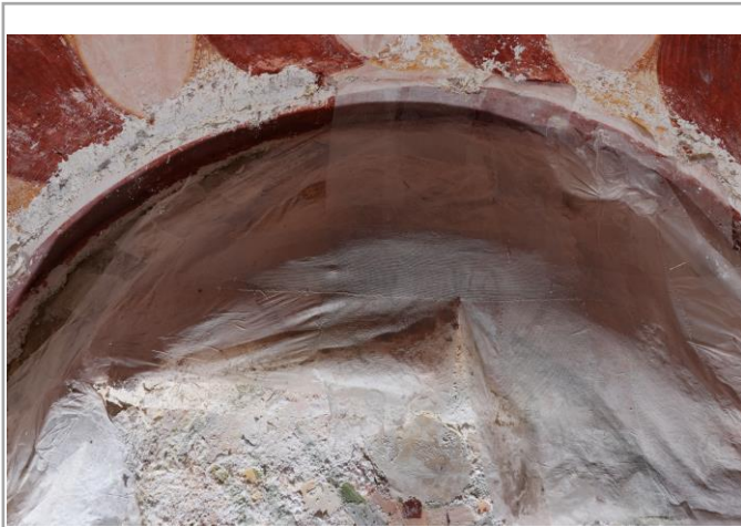
Two months after reinforcement. May 2024
